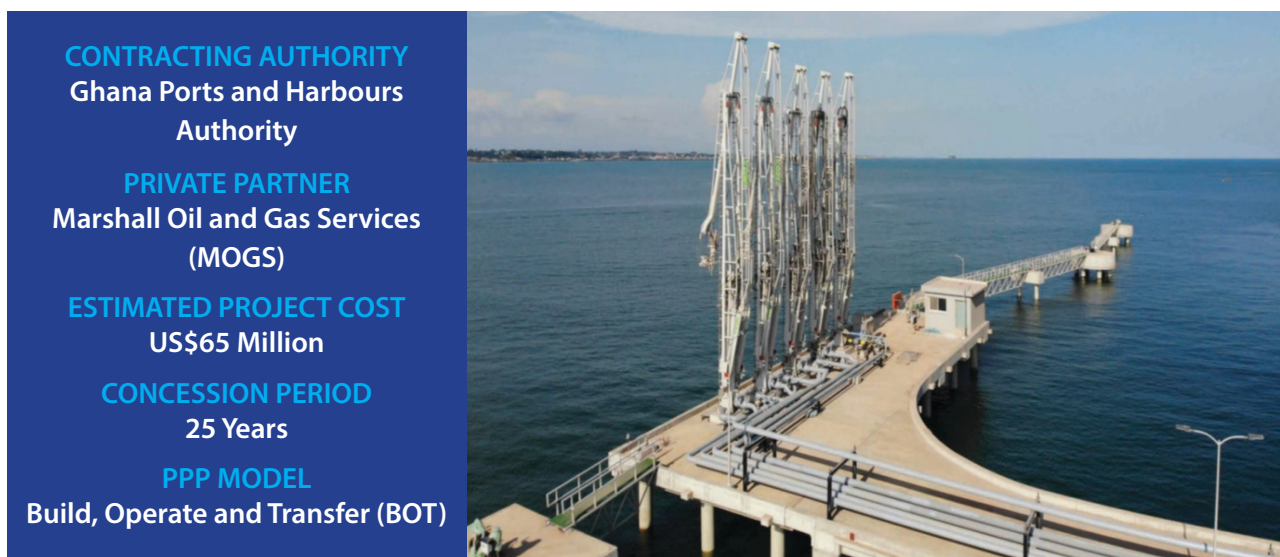
Figure 24: Loading Arms Dolphins installed at the Takoradi Liquid Bulk Terminal
