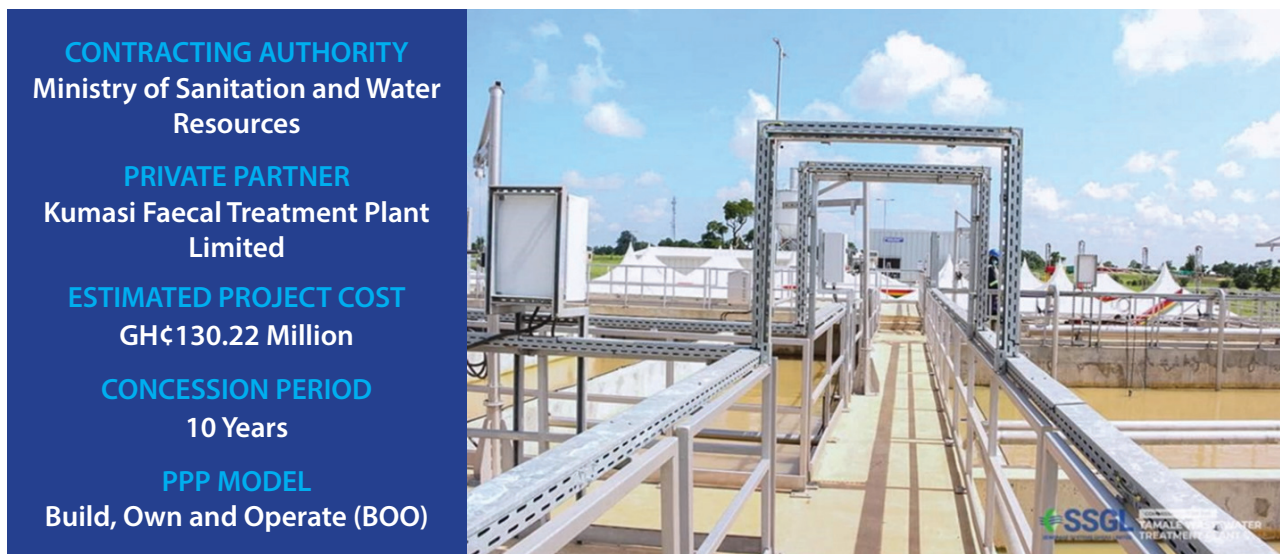
Figure 15: Installation of the Liquid Waste Treatment Plant
