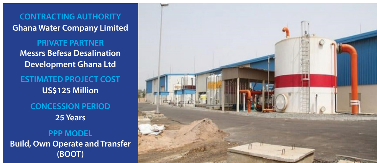
Figure 16: Teshie Nungua Desalination Plant
