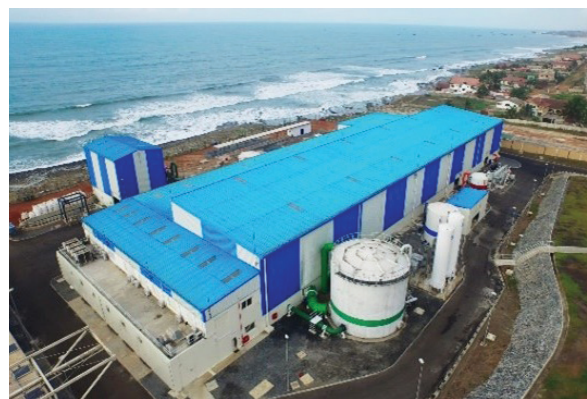
Teshie Nungua Desalination Plant
