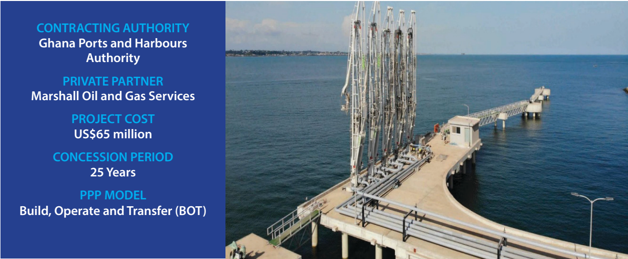
Figure 13: Loading Arms Dolphins installed at the Takoradi Liquid Bulk Terminal
