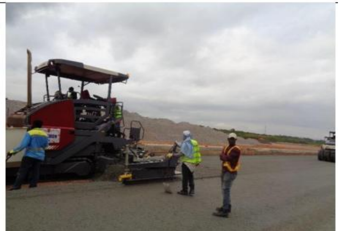
Laying of CBGM Base (First layer) at Terminal
