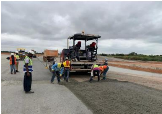
Laying of CBGM Base (First layer) at Terminal
