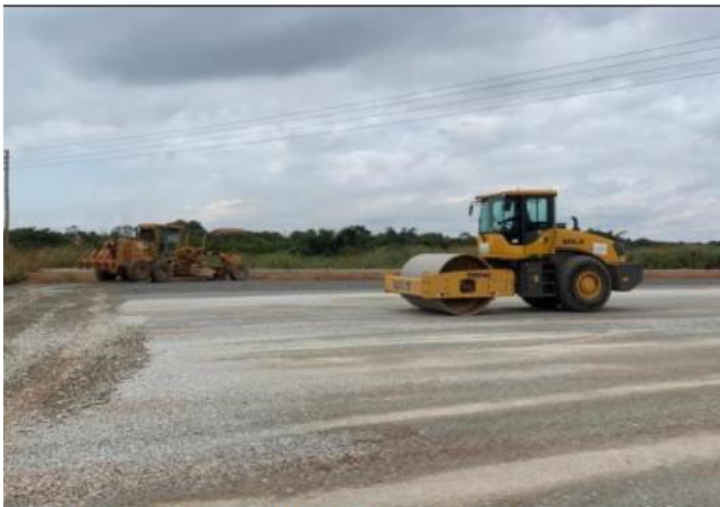
Laying & spreading of sub-base (Terminal)
