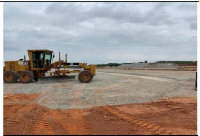
Laying & spreading of sub-base (Terminal)
