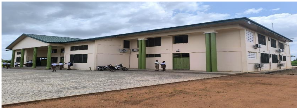
Completed dining hall at Ho School of Hygiene
