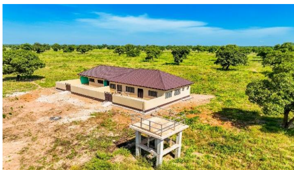
Completed CHPS Compound at Kparigu
