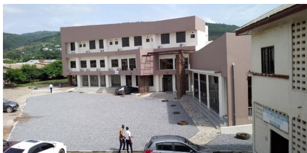
Construction of Business Resource Centre With Restaurant, Conference Hall, And Hostel Facility At Lower Manya Krobo
