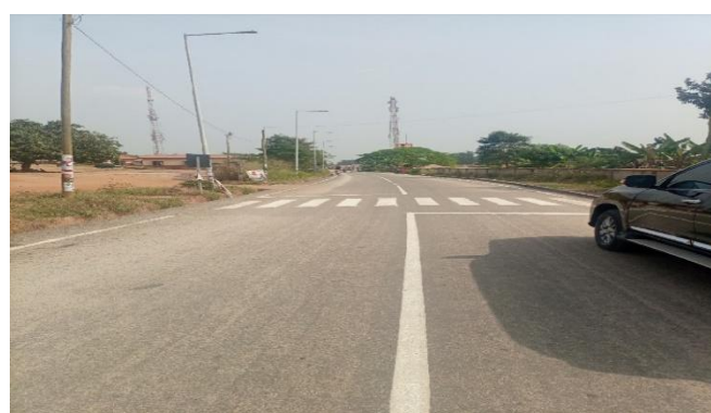
Rehabilitation of Kyerapatre Old Town Road Phase One (1.0km) at Asokwa
