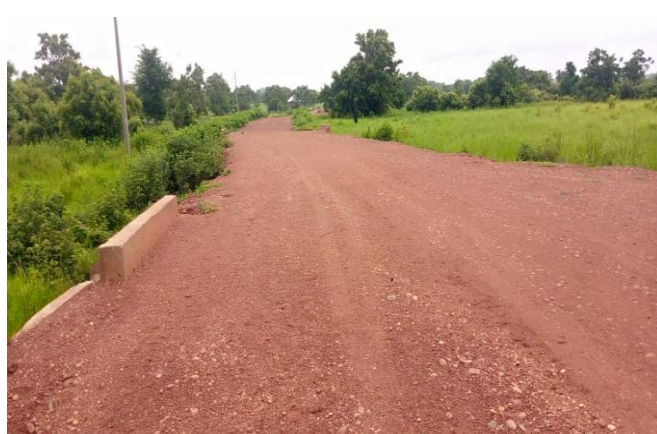
Culvert at Yamo-Karaga-Kpalguma, Northern Region
