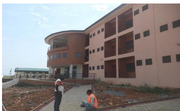
Construction Of 3-storey 44 Rooms Hostel at Greenery Site at Kibi
