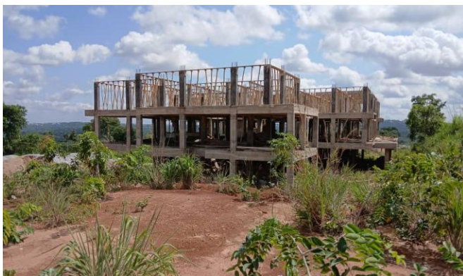
Ongoing 3-storey 12-unit Block of Flats for Ahafo Regional Police Command, Goaso.
