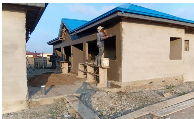
Construction of four (4) Unit Teachers Quarters and a Mechanized Borehole at Adjei-Kojo TWMA Basic Schools, Tema West District, G. Accra Region
