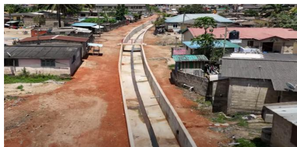
Construction Of Storm Drain From Obiri Junction To Mempeasem - Sofon Zongo (400m Long) At Effia
