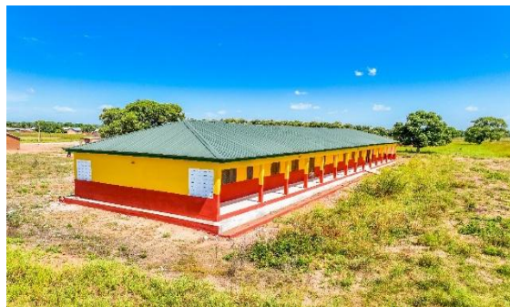
Completed 3Unit Classroom Block at Nabulugu
