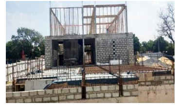
19% completion Expected to be completed 2 nd quarter 2024
