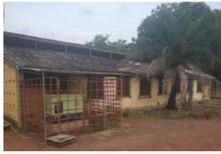
Office Accommodation before 2016
