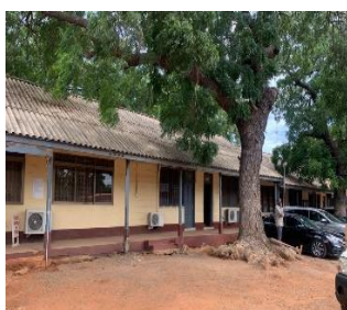
Old LC Greater Accra Regional Offices
