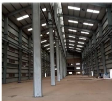
Fabricated Steel Structure
