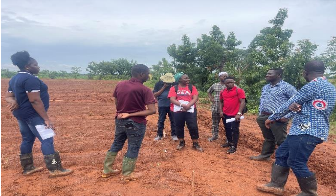
NBA officials undertaking a CFT monitoring and inspection at a site in Nyankpala.
