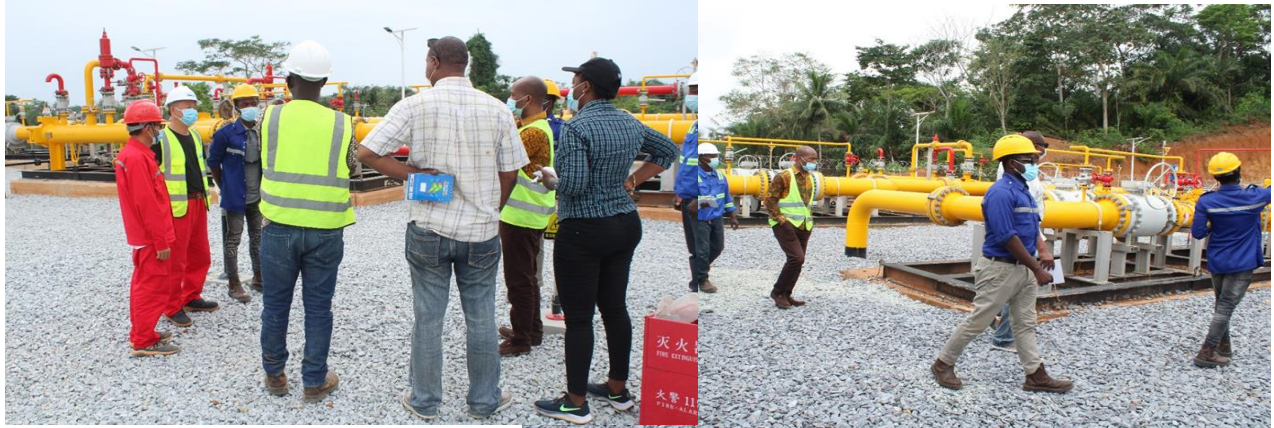
Monitoring of Ghana Gas Atuabo Plant
