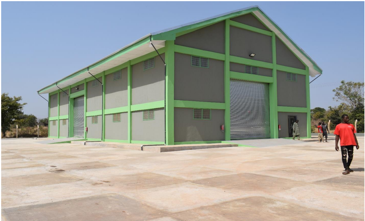
Main warehouse at Hain in Upper West Region
