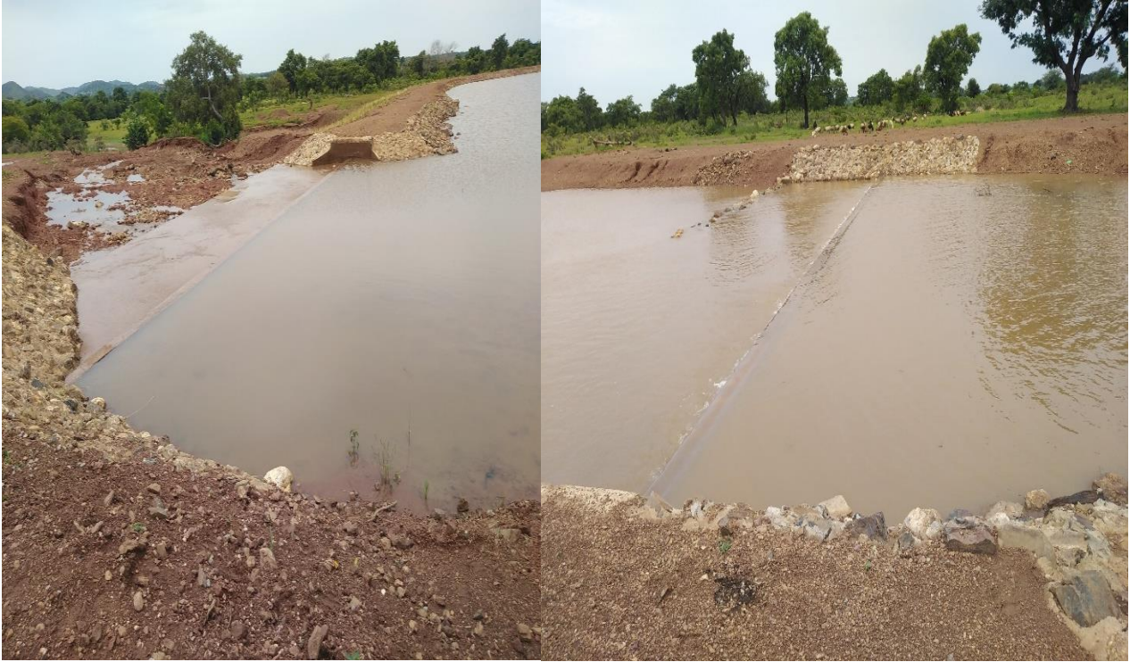
Spillways of Small Earth Dam at Namolgu in the Upper East Region
