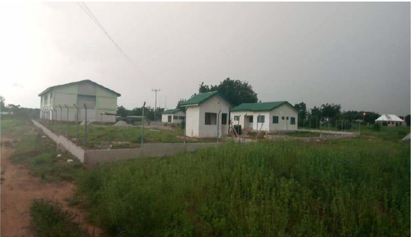
Completed warehouse with ancillary structures at Bole in Savannah Region
