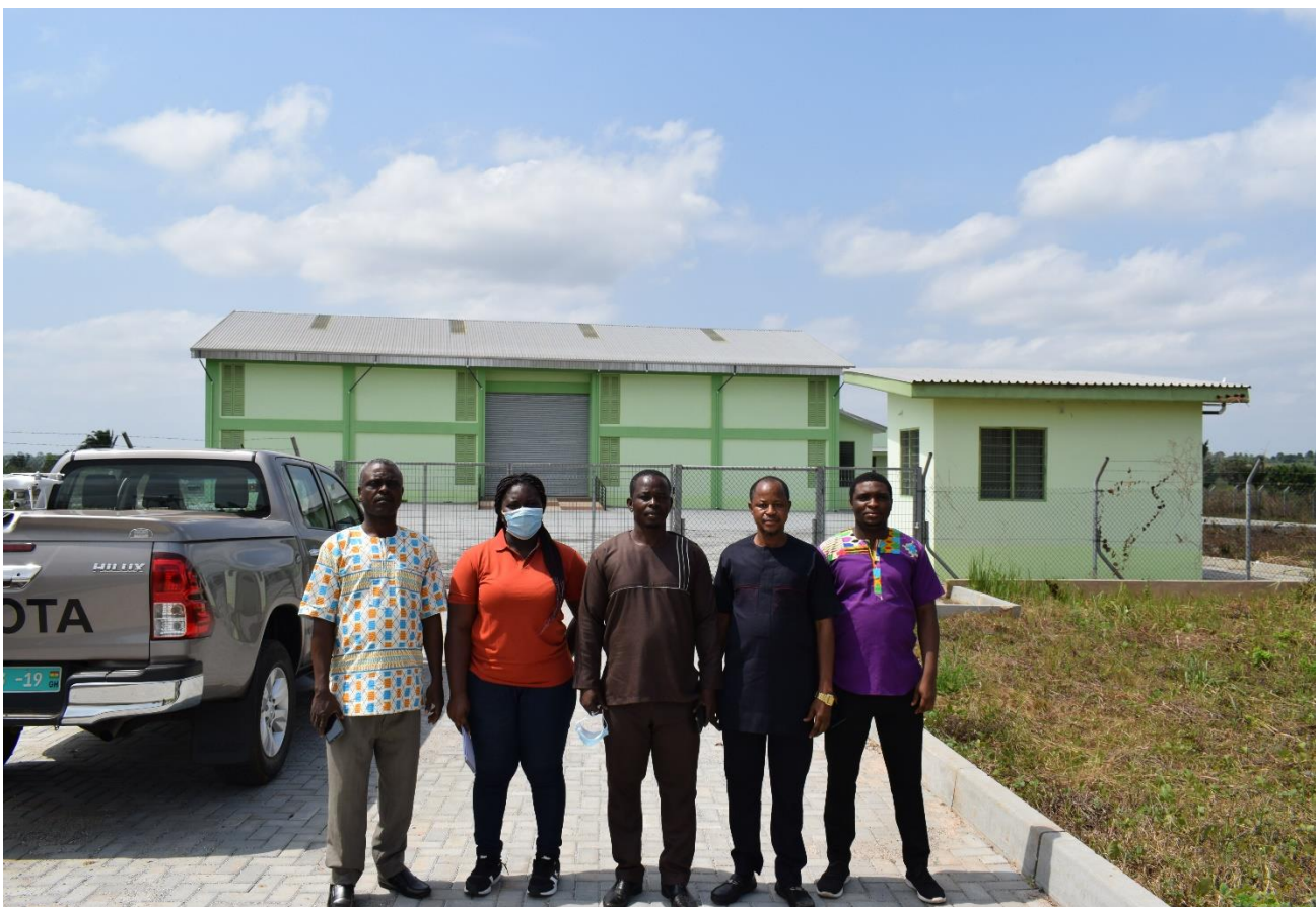
Monitoring Team at completed warehouse with ancillary structures- Dzodze in Volta Region
