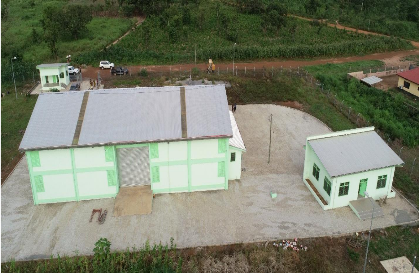
Completed warehouse with ancillary structures at Chinderi in Oti Region
