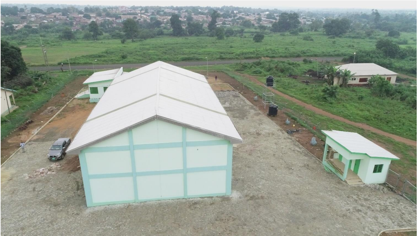
Completed warehouse with ancillary structures at Nkwanta in Oti Region
