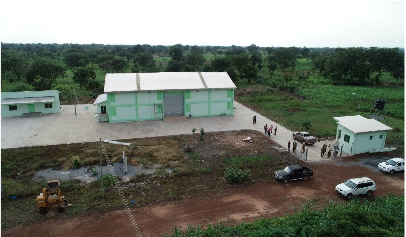
Completed warehouse with ancillary structures at Chinderi in Oti Region
