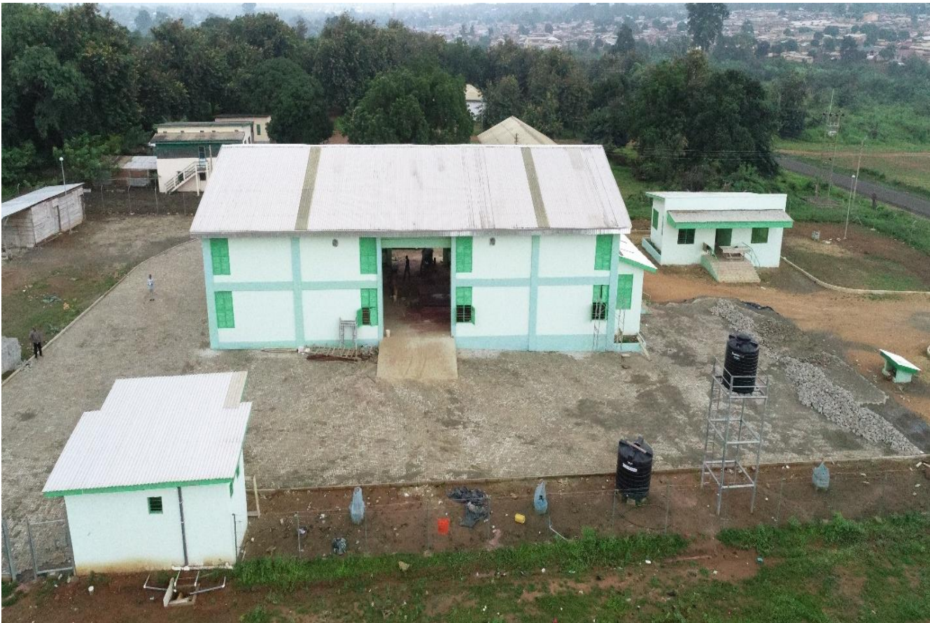
Completed warehouse with ancillary structures at Nkwanta in Oti Region
