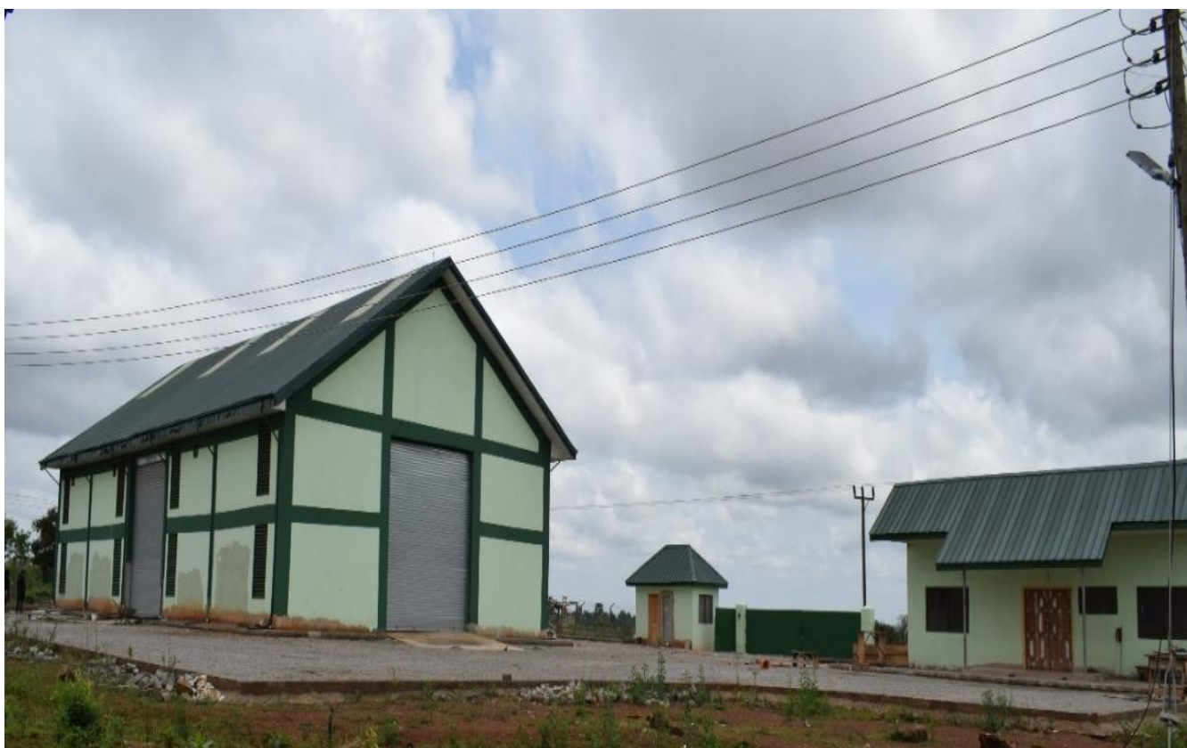
Completed warehouse with ancillary structures at Nkranza in Bono East Region
