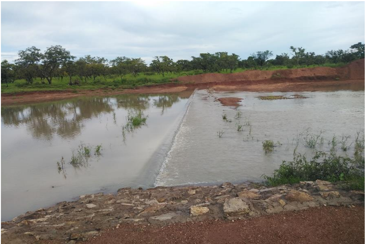
Spilling of completed Small Earth Dam at Duong in the Upper West Region
