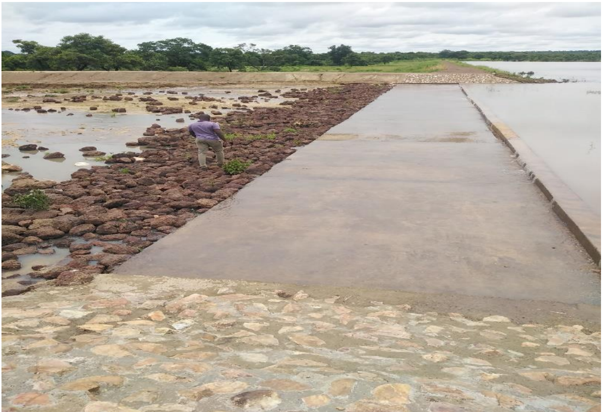
Spilling of completed Small Earth Dam at Kataa in the Upper West Region
