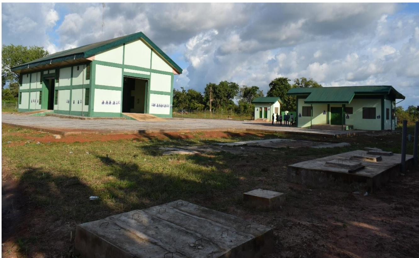
Completed warehouse with ancillary structures at Kwame Danso in Bono East Region
