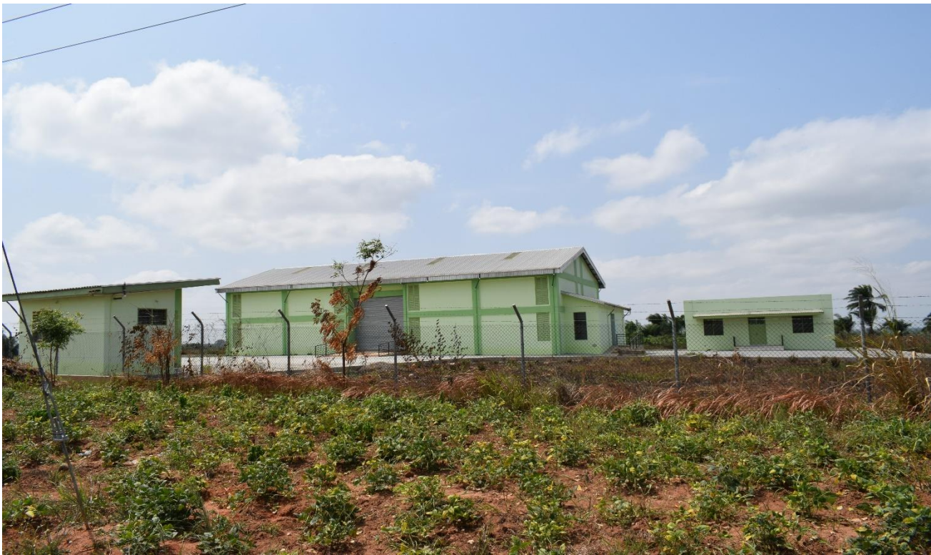
Completed warehouse with ancillary structures at Dzodze in Volta Region
