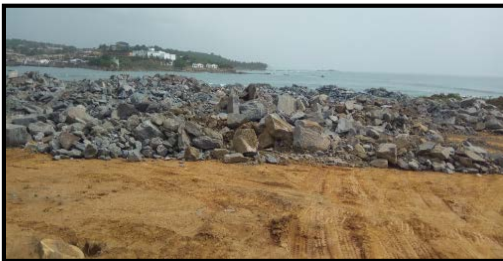
Figure 5: Dixcove Sea Defence Project
