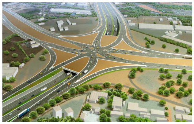
After Completion Impression - Tema Motorway Roundabout after Completion
