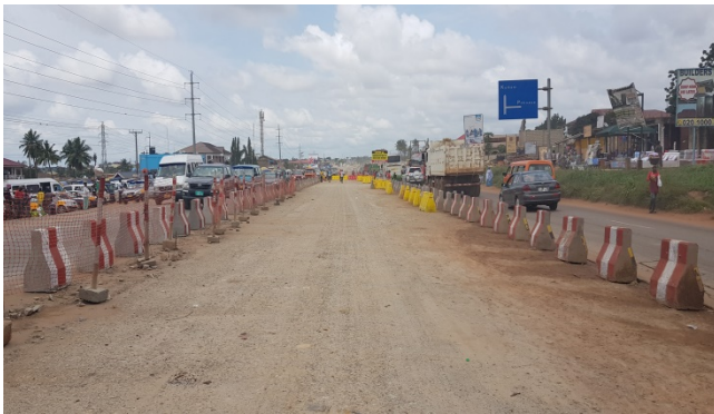
Ongoing Works – Pokuase Interchange Project
