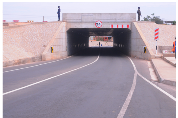
After Completion - Spintex Road – East Legon Tunnel
