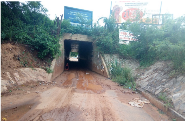
Before Situation - Spintex Road – East Legon Tunnel
