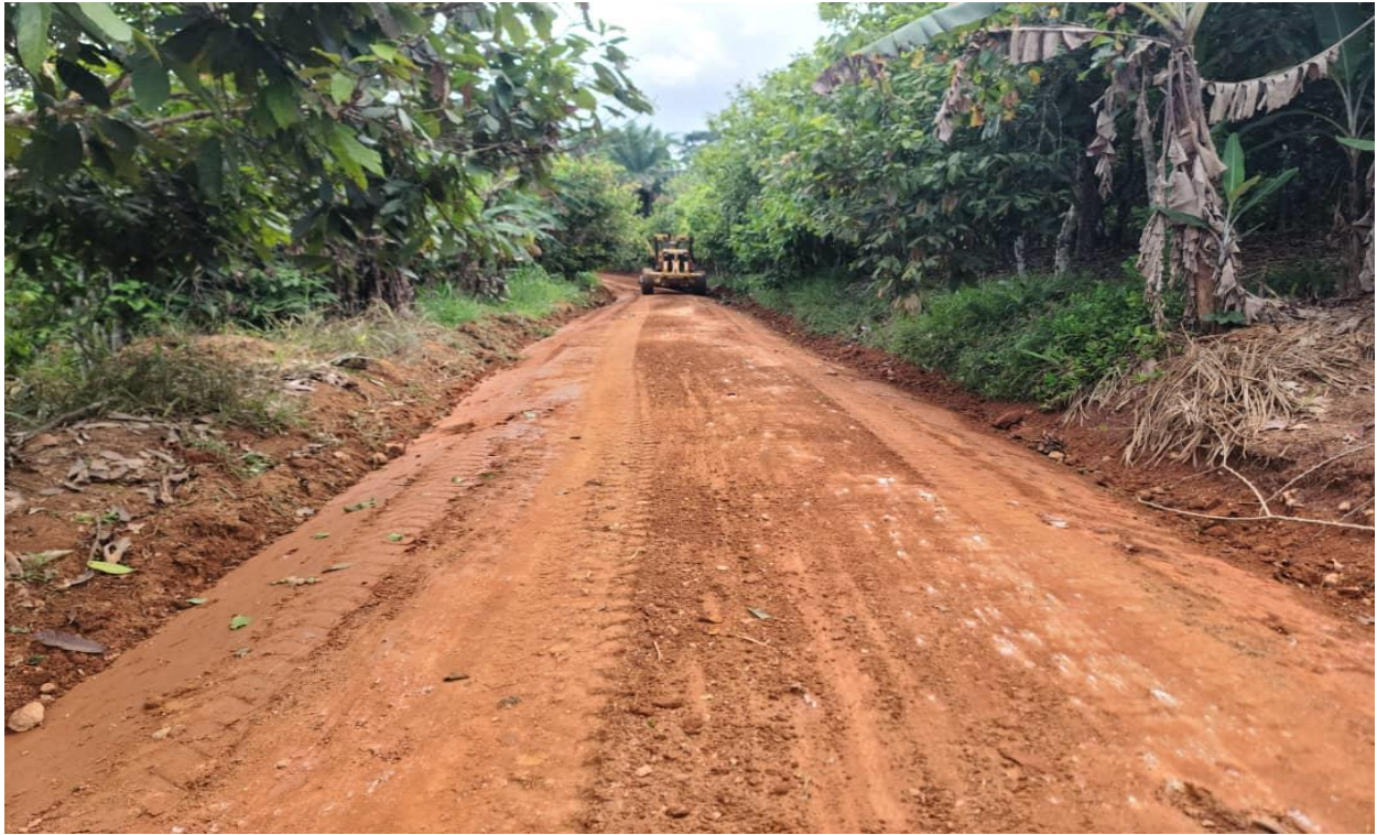
Reshaped 13.1km feeder roads
