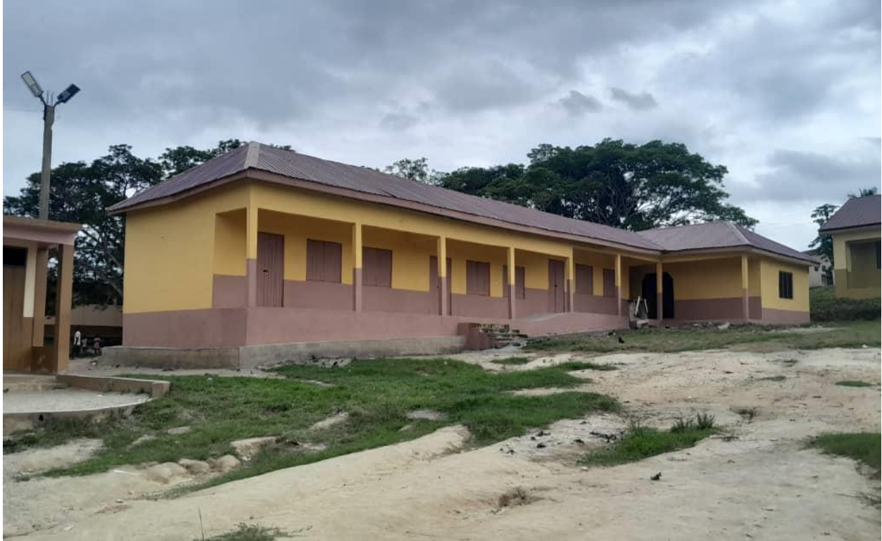
COMPLETED 3-UNIT CLASSROOM BLOCK AT ASSORKO
