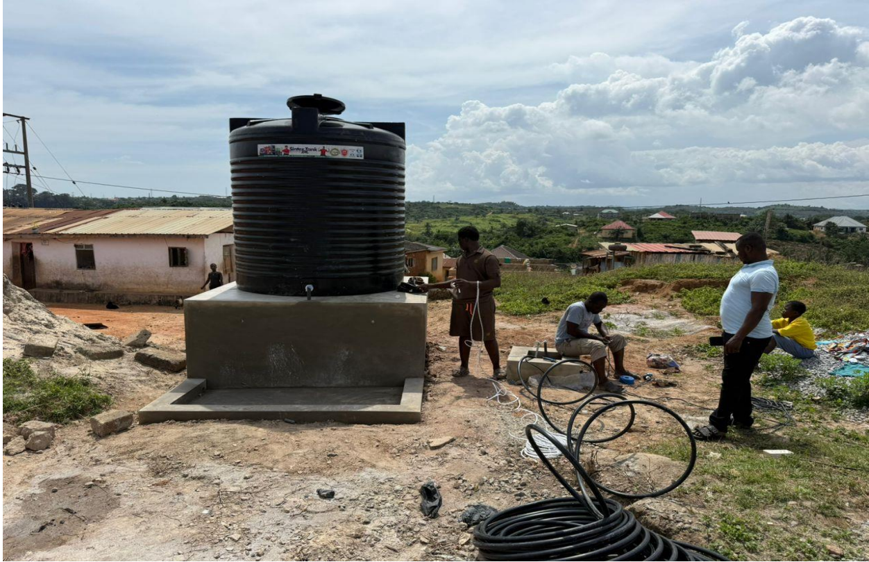
CONSTRUCTED AND MECHANISED OF BOREHOLE AT ASEMASA NO. 2
