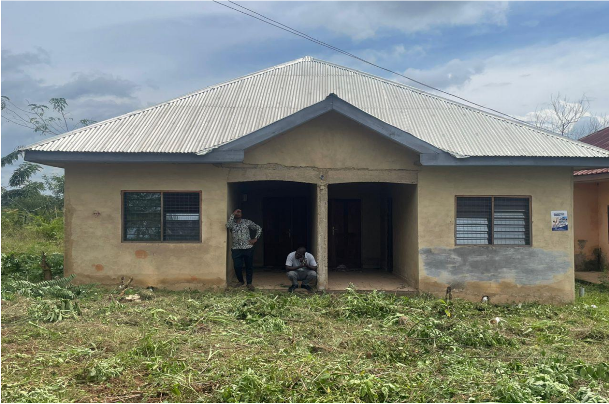
Completed 1No 2Unit Semi-Detached Nurses Quarters-Dadieso
