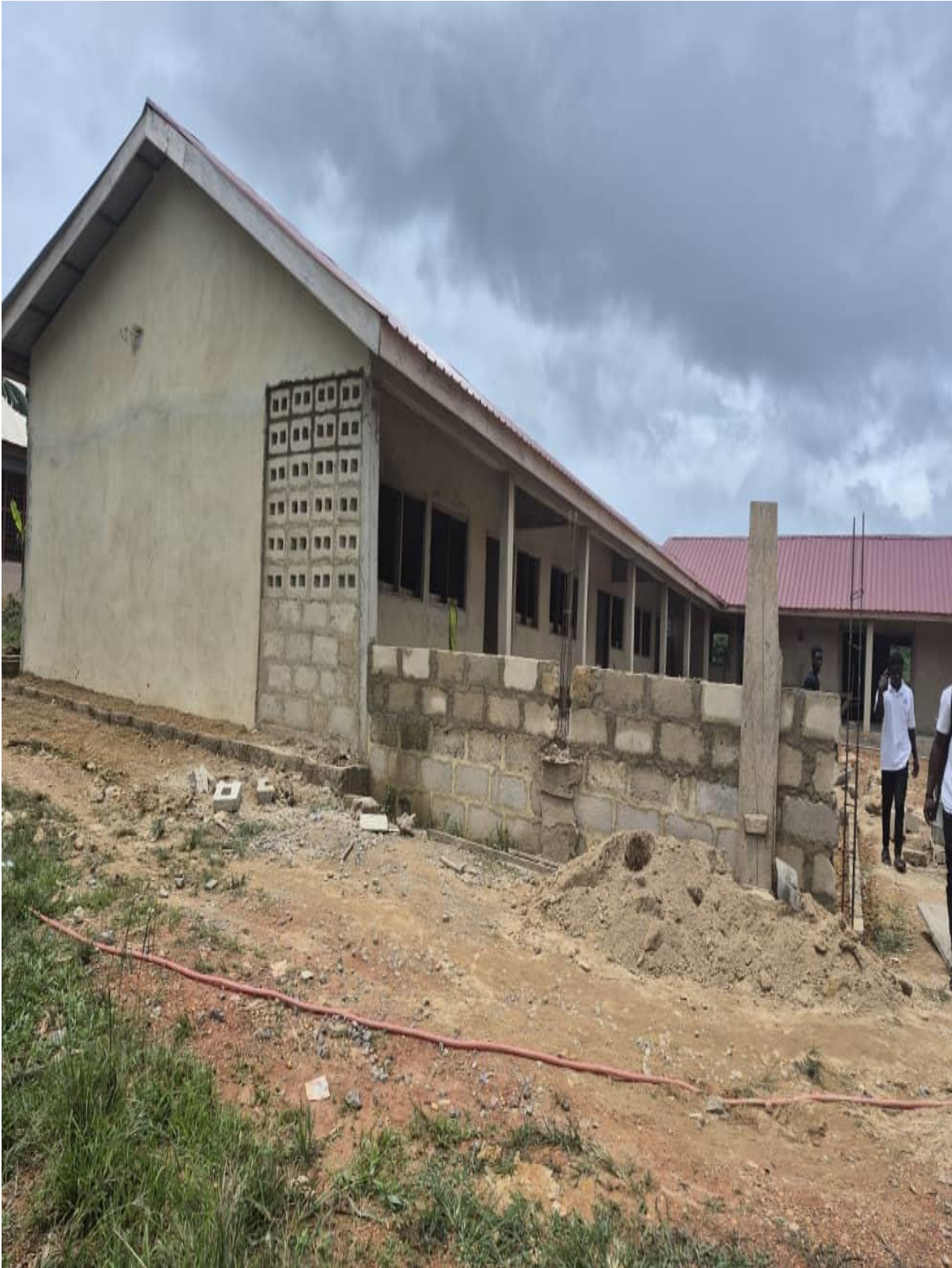
Completed 6Unit Classroom Block at Asuapokua
