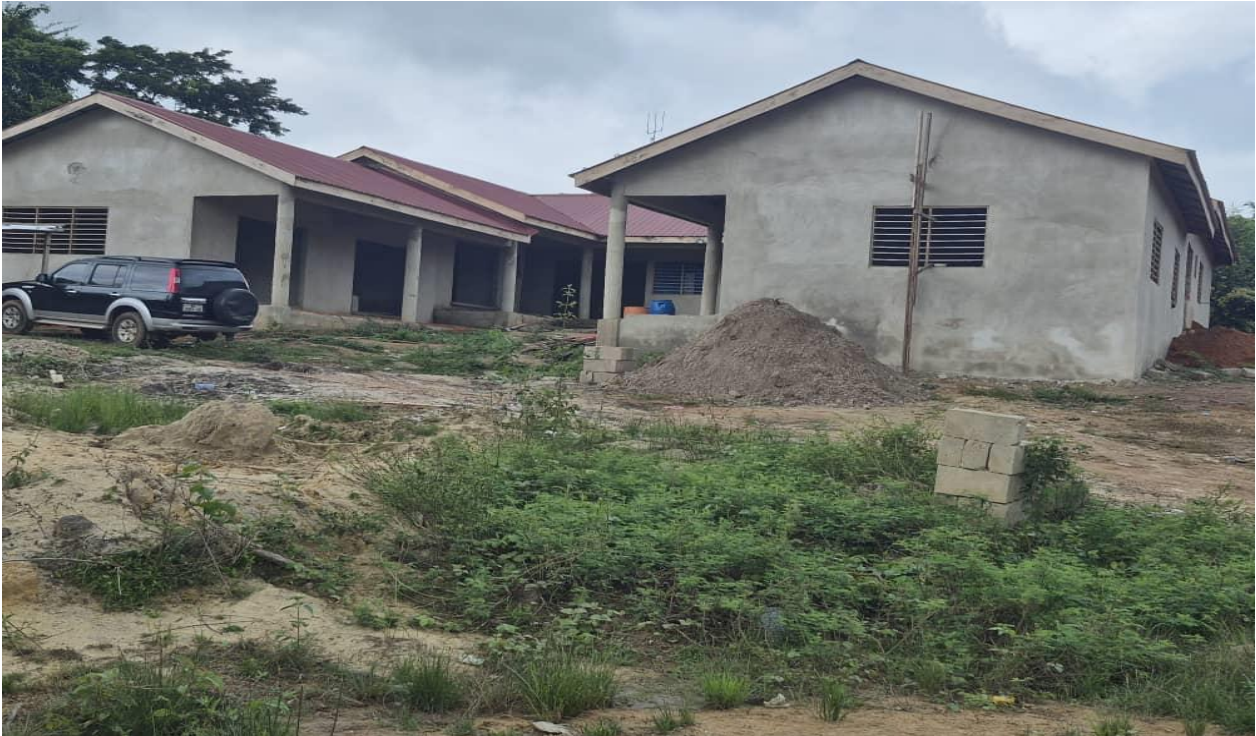
Completed of PWD Workshop at Karlo
