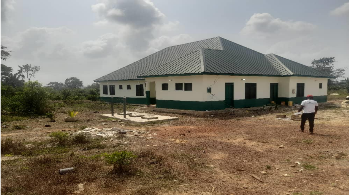
Completed 1No CHPs Compound and 1No. Nurses Quarters with Borehole at Adiepena
