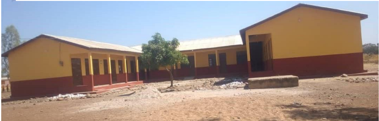
Rehabilitated 6-unit classroom block at Dagliga-SOCO
