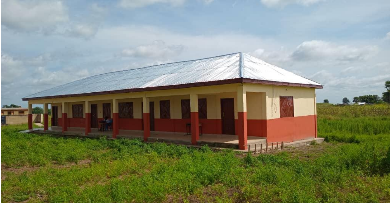
Constructed 3-unit classroom block with head teachers' office and a store at Soliga DACF-MP.
