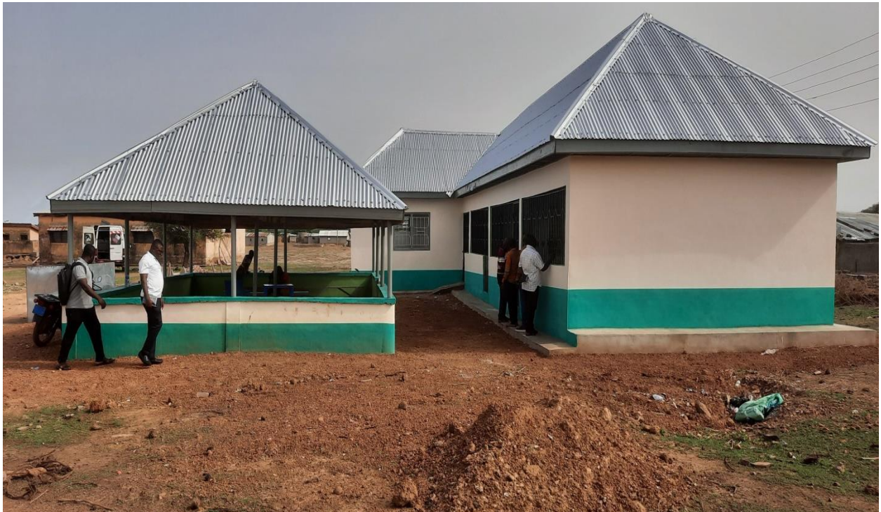
Constructed and renovated Kadema CHPS compound under SOCO
