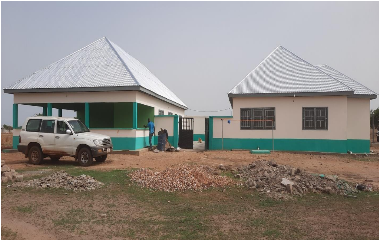
Constructed 1No CHPS compound with ancillary facilities at Yimonsa under SOCO
