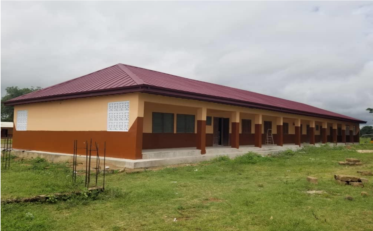
Constructed and furnished 3-Unit Classroom block with 4-seater KVIP Toilet at Kantia
