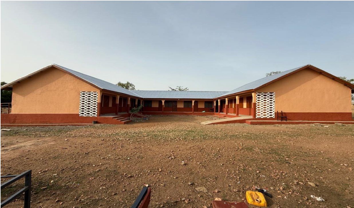
Rehabilitated 6-Unit Classroom Block at Gambibgo
