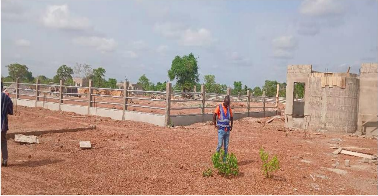
Construction of animal market at Busunu
