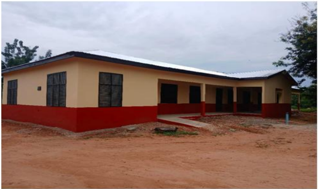
1 no. 3 unit classroom block constructed at Kurabaso
