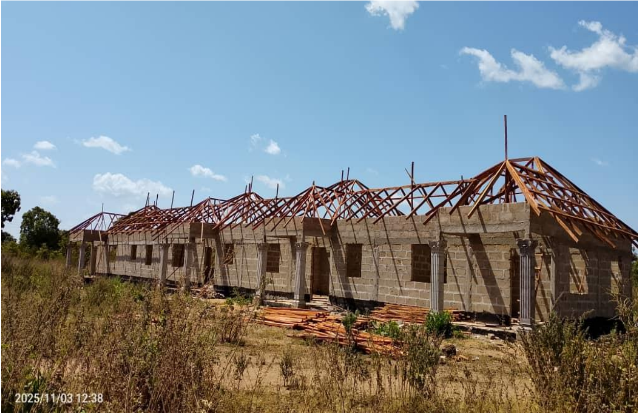
Construction of 1NO.Studio Apartment for Teachers at Daboya-Ongoing
