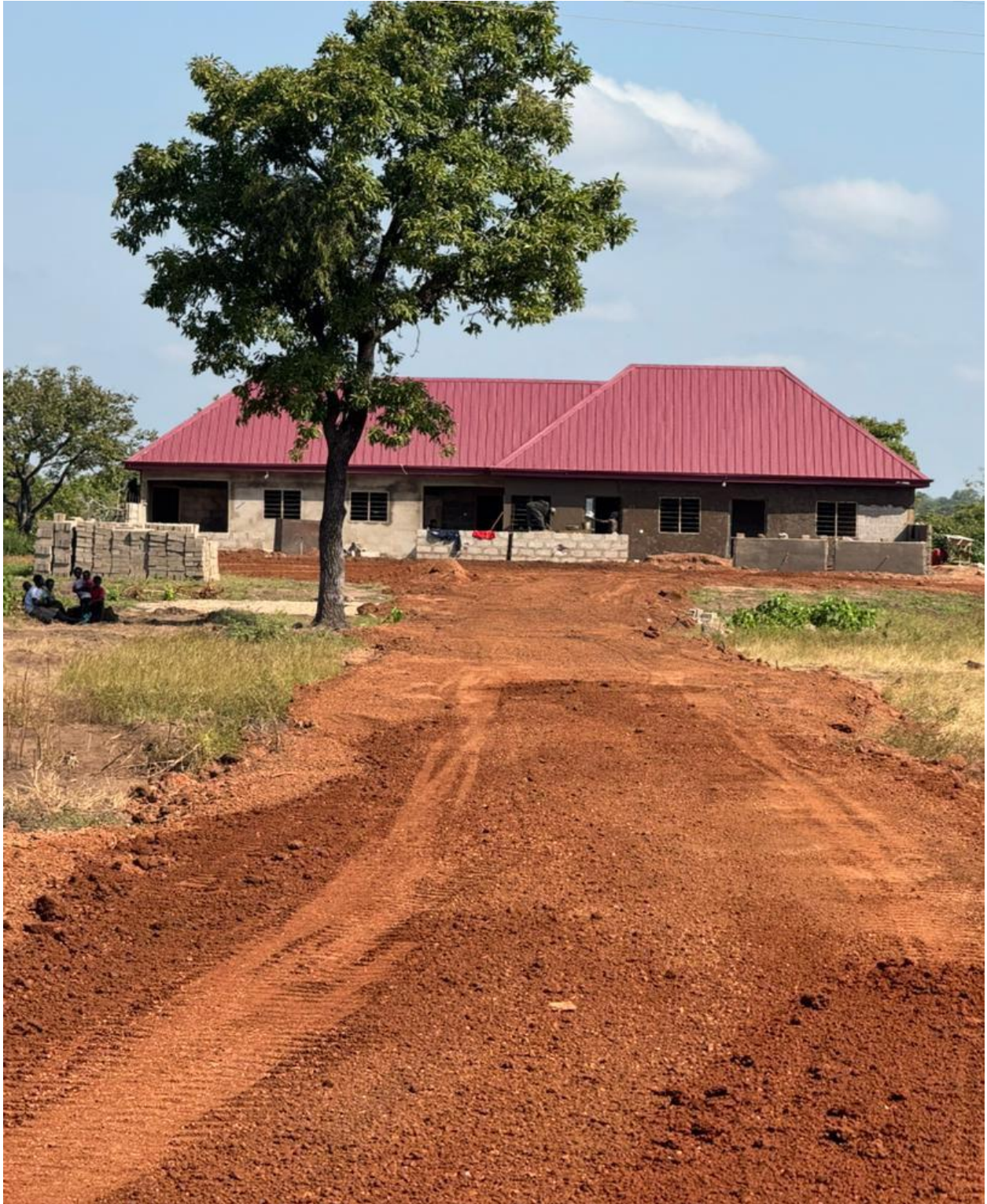
Construction of CHPS at Kakoshie
