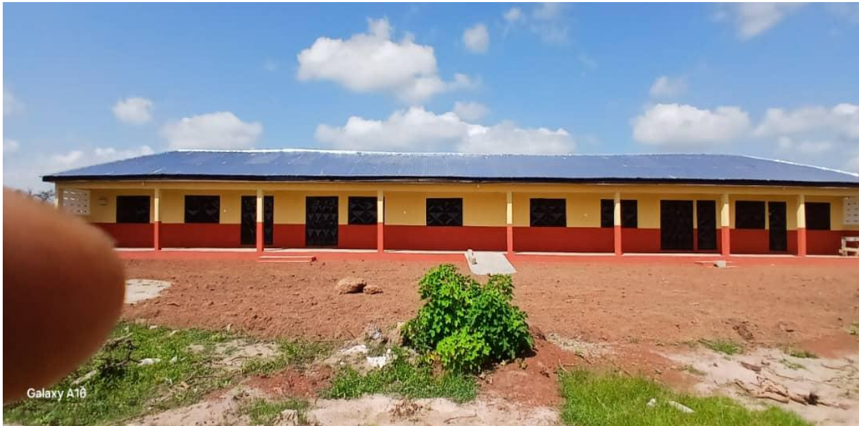
Constructed 1 no. 3 unit classroom block at Matilapor
