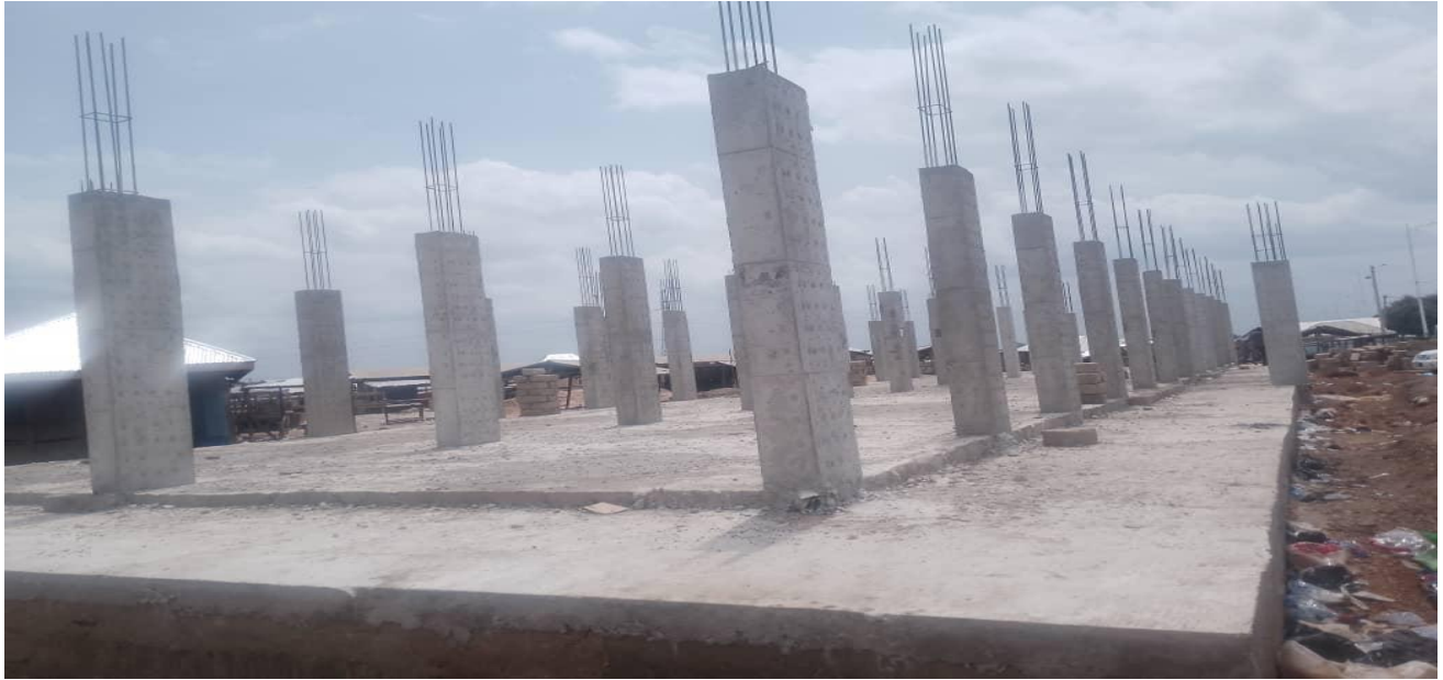
Construction of 1no. 2 story, 40 unit lockable stores at Buipe
