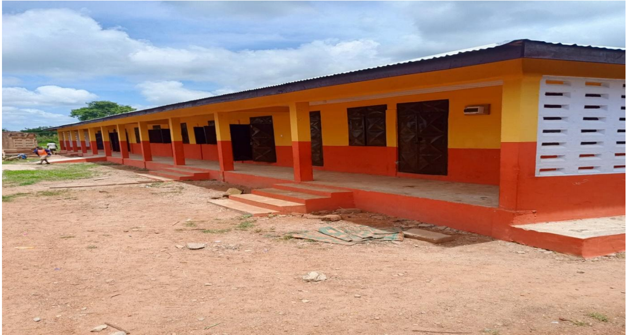
Constructed 1no. 3 unit classroom block with ancillary at Fufulso
