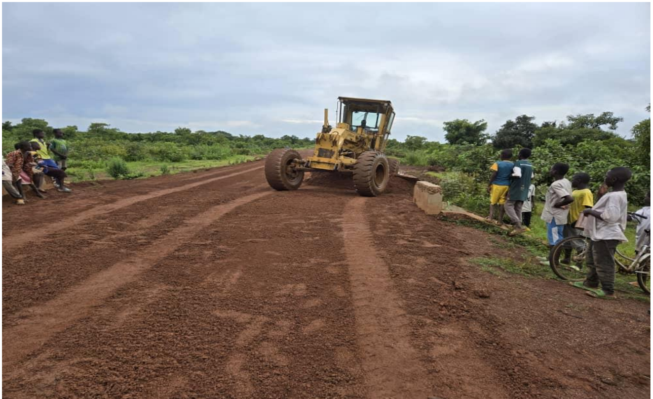
Rehabilitated Kusawgu-Tulwe feeder road. (63kms)
