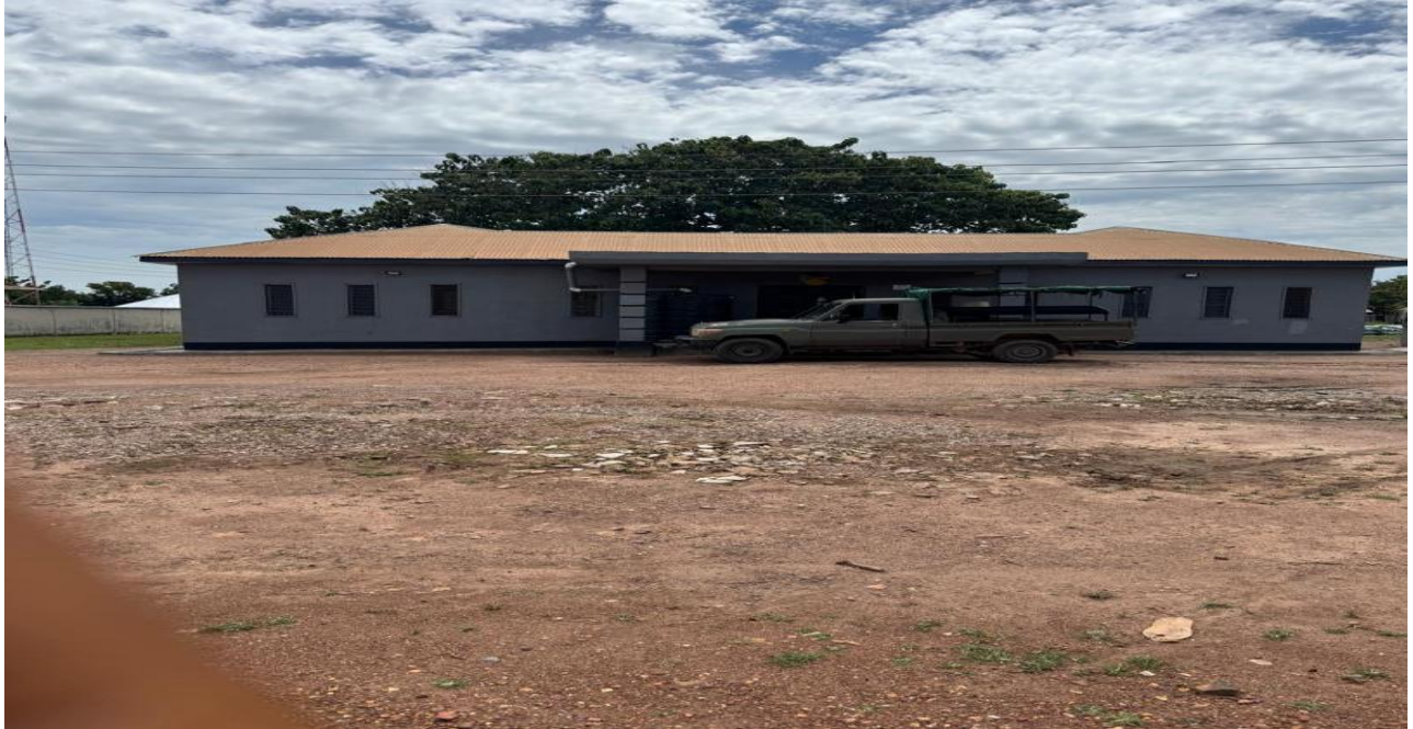
Rehabilitated military accommodation at Buipe.
