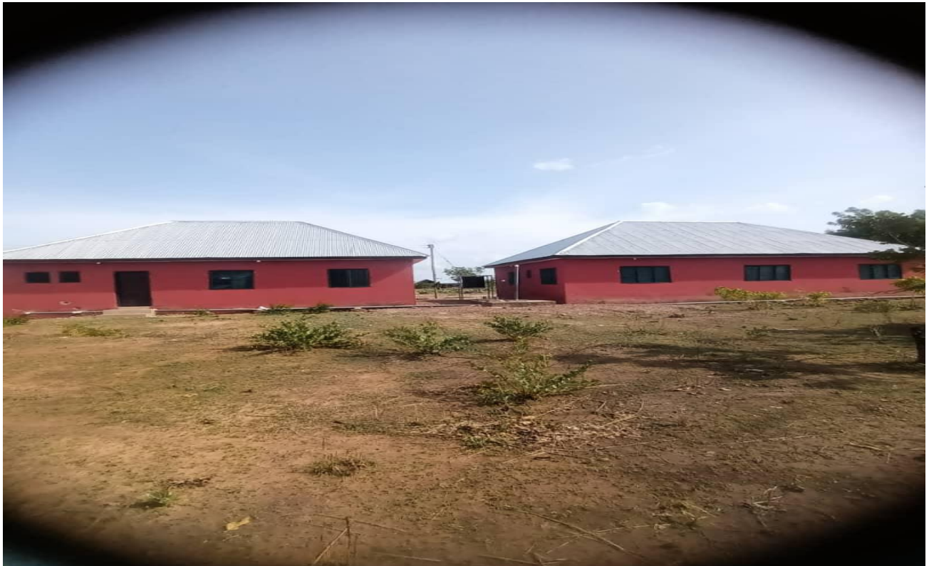
Constructed 1no. CHPS compound, 3-unit 1 bedroom semi-detached
