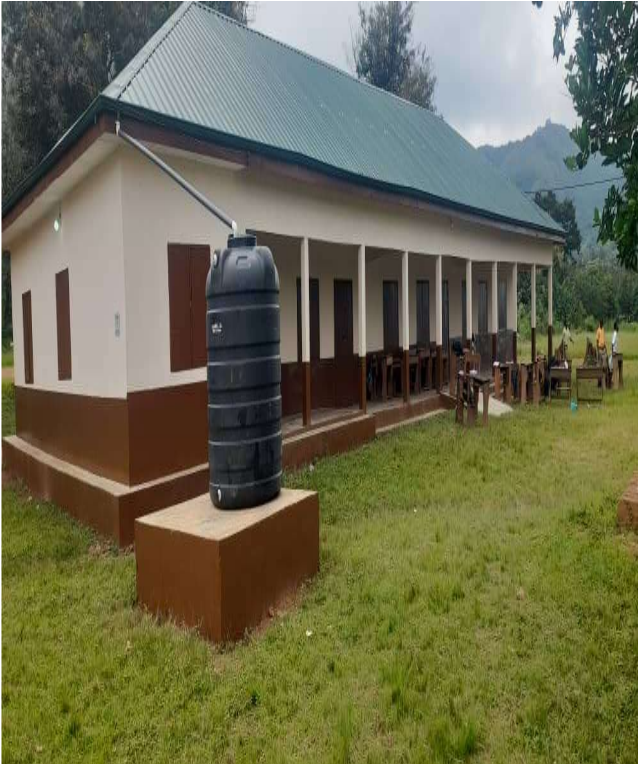
REHABILITATION OF RC. JHS AT LIKPE MATE
