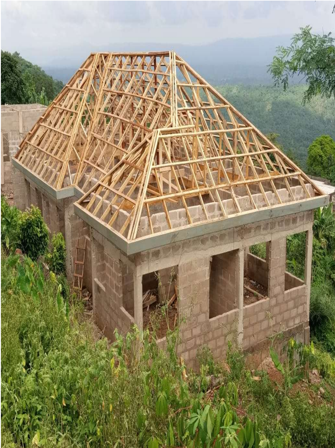
CONSTRUCTION OF CHPS COMPOUND AT AKPAFU TODZI
