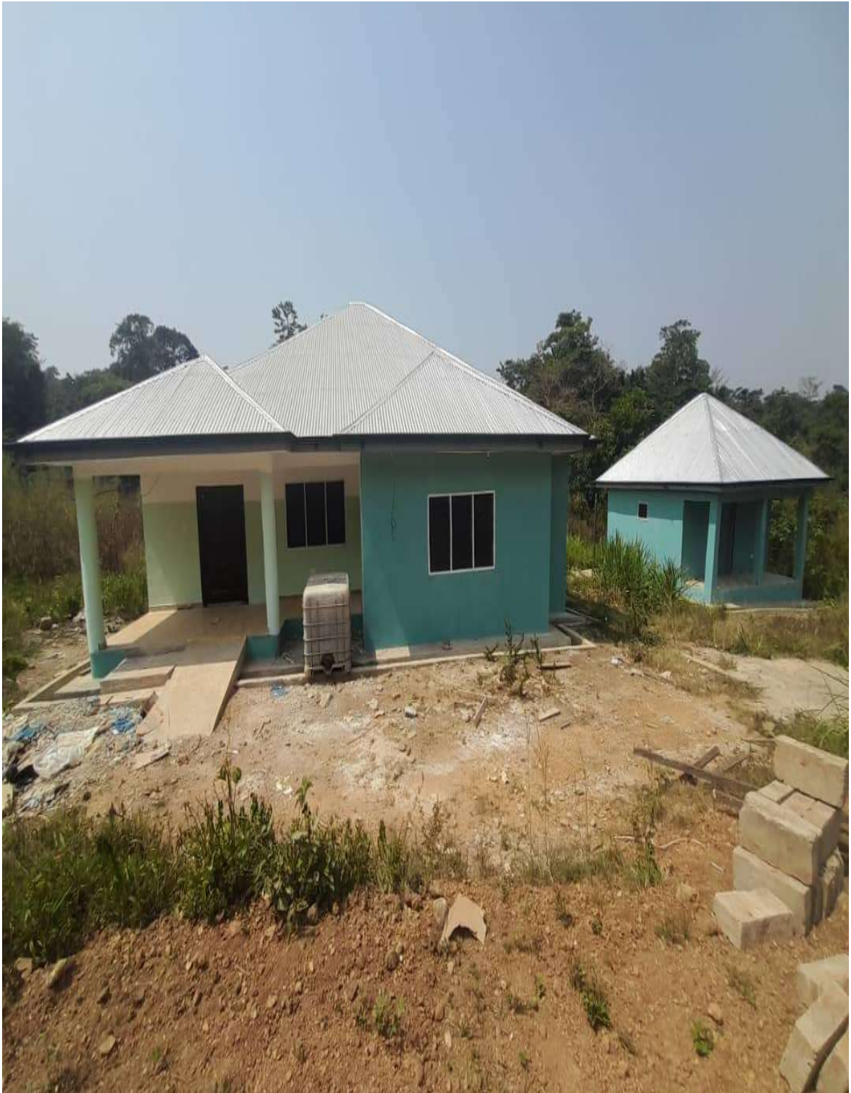
CONSTRUCTION OF HEALTH DIRECTOR, s BUNGALOW AT LIKPE MATE
