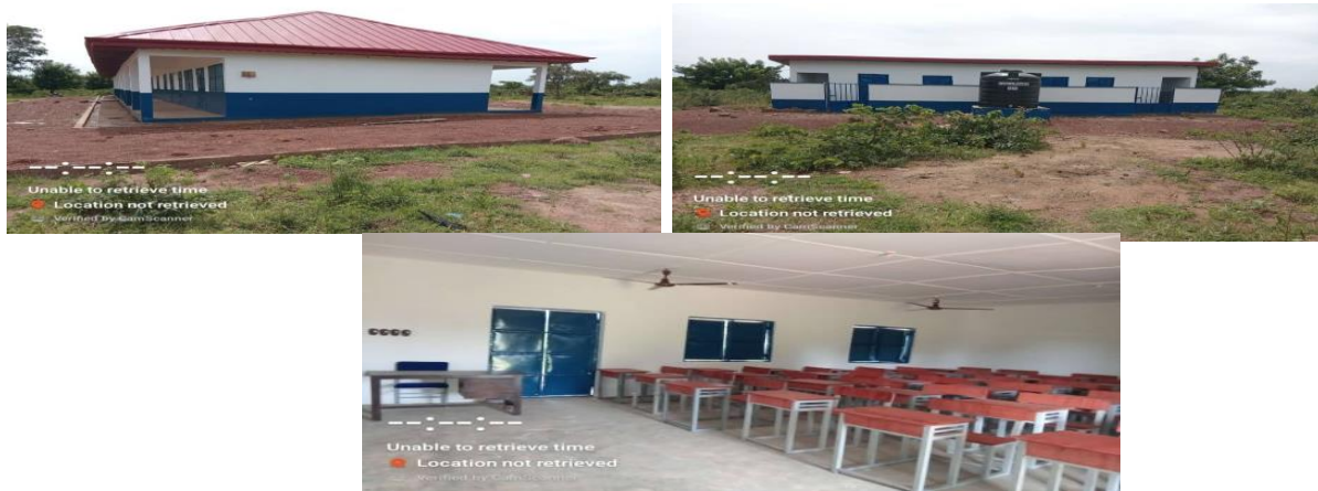
Key Achievements in picture Completed and furnished 3 -Uits Classroom Block at Bini
