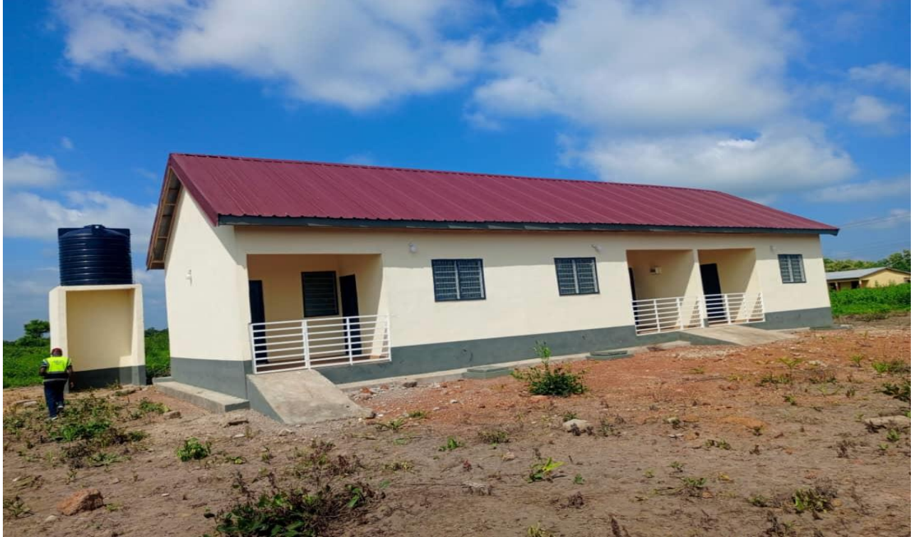
CONSTRUCTED NURSES QUARTERS AT BULKPALI FUNDED BY SOCO
