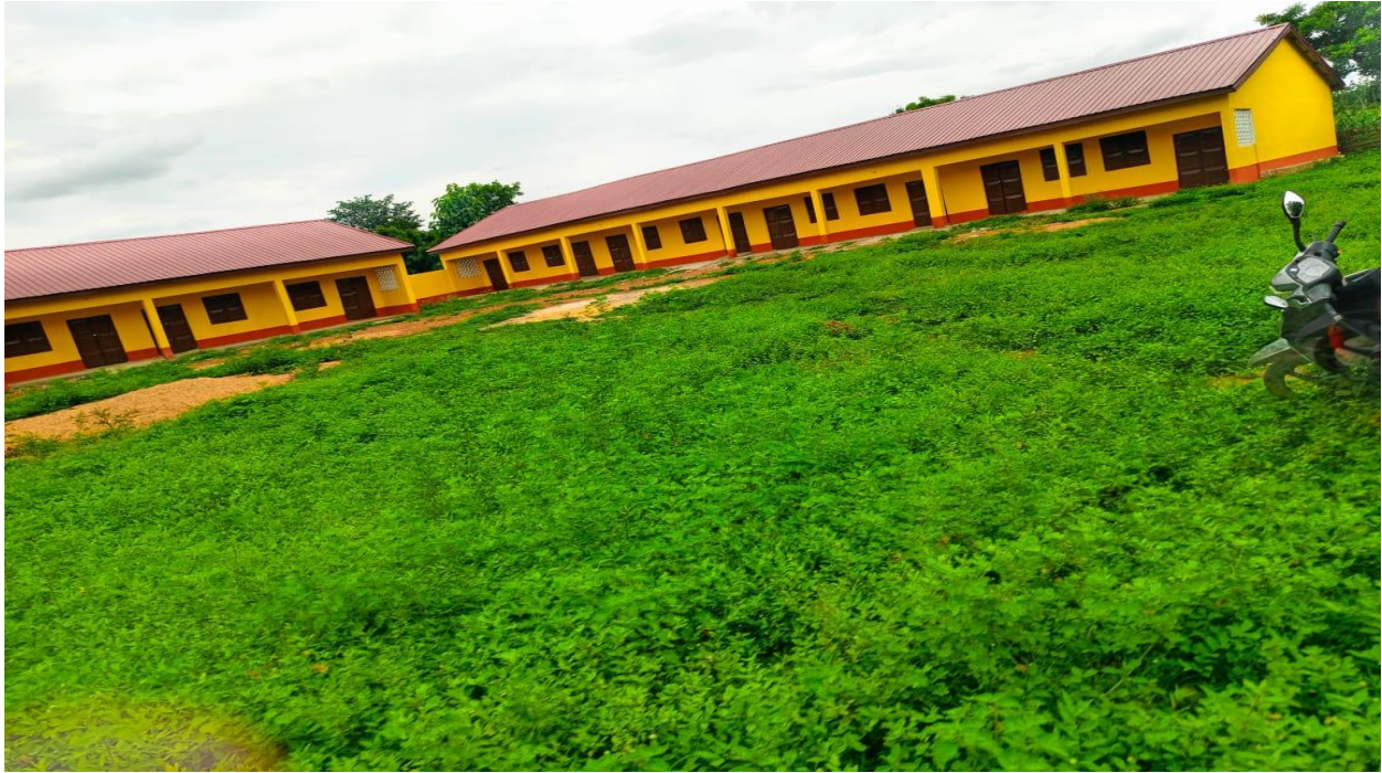
CONSTRUCTED 1NO. 6-UNIT CLASSROOM BLOCK AT NAKPALI BORLE FUNDED BY SOCO
