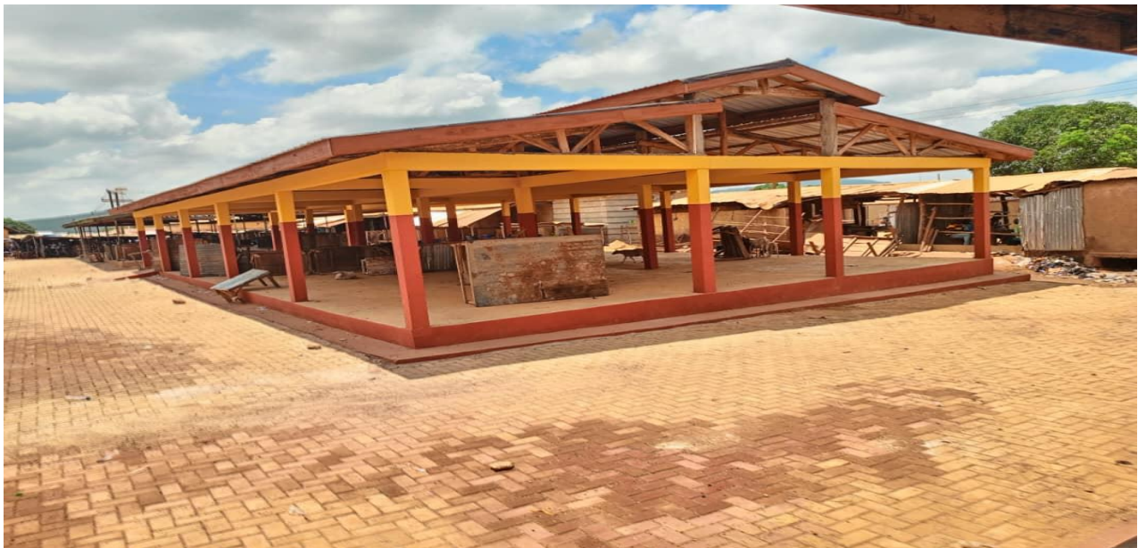
RENOVATED TATALE MARKET SHED FUNDED BY SOCO
