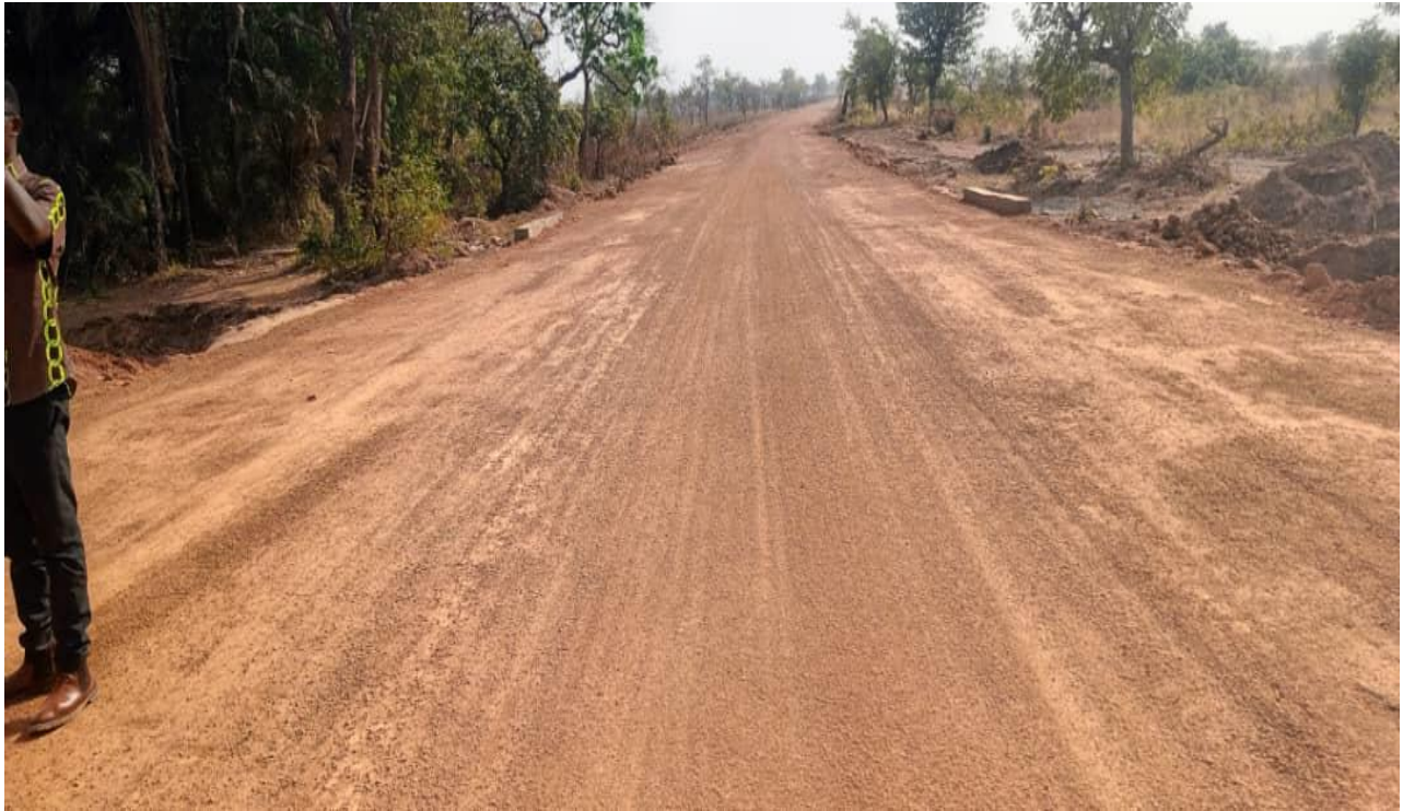
CONSTRUCTED 7KM SHEINI-DAPROBA FEEDER ROAD FUNDED BY SOCO
