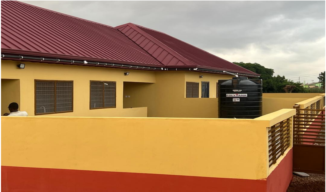
Above: CHPS Compound and Accommodation constructed at Kunyevella Community.
