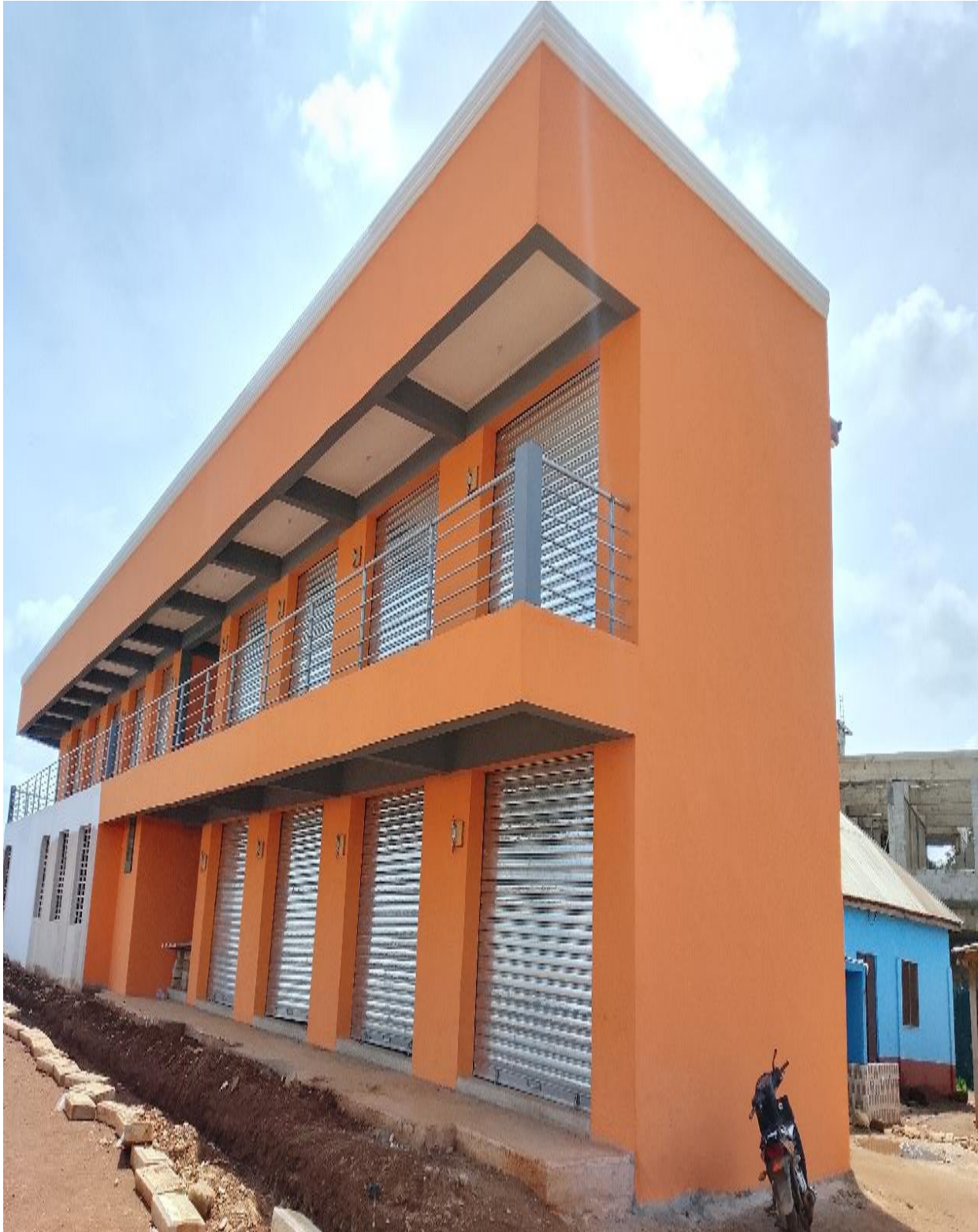
Above: 24 No. Lockable Stores constructed at Kalpohin
