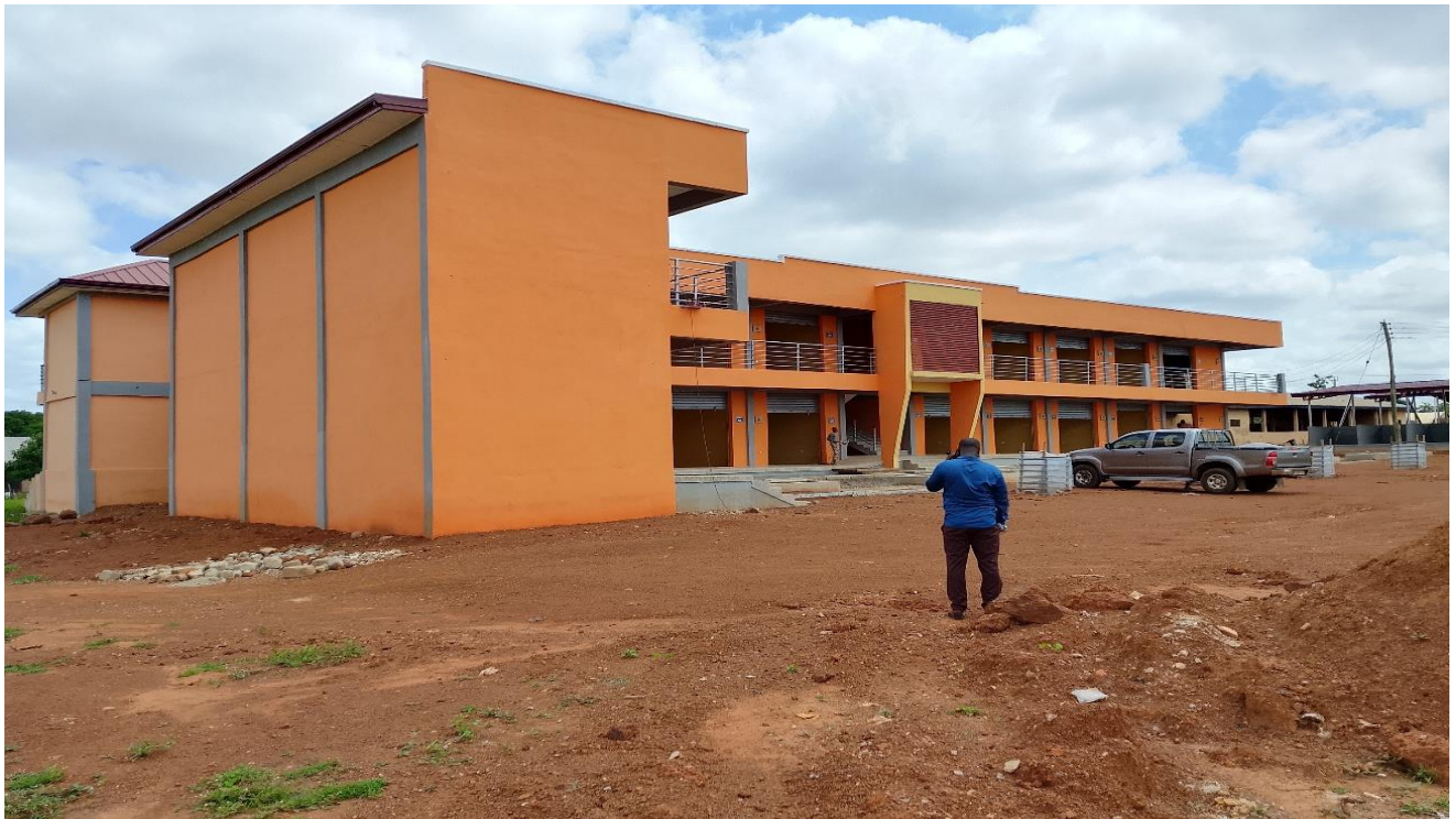
Above: 24 No. Lockable Stores constructed at Sagnarigu Market
