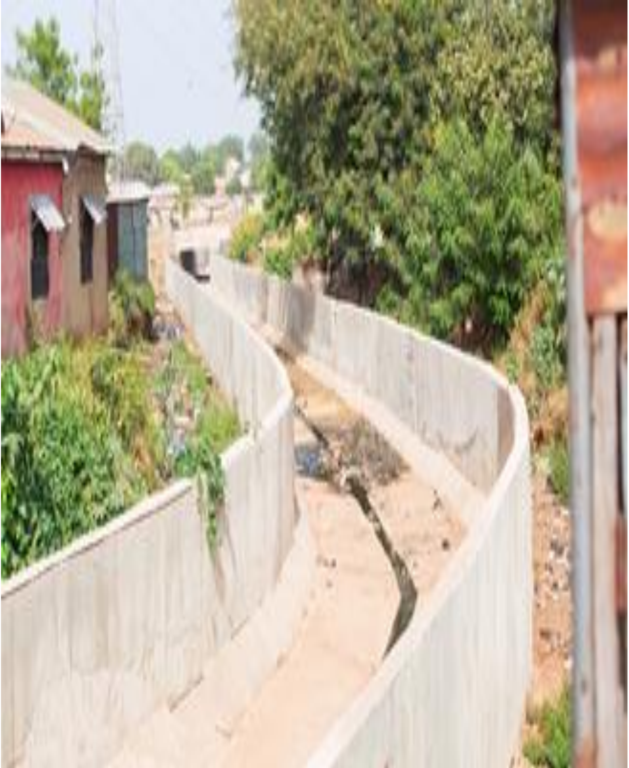
Above: Nobisco-Naluro drain constructed
