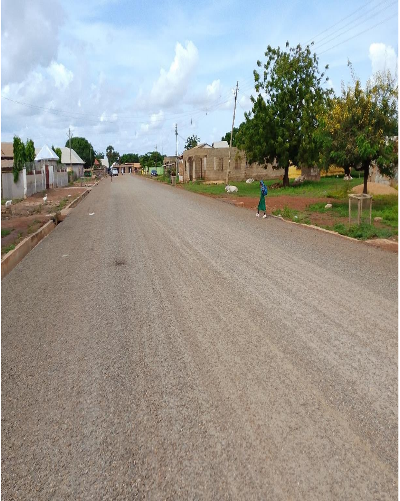
Above: Kpalsi- Dimala road constructed
