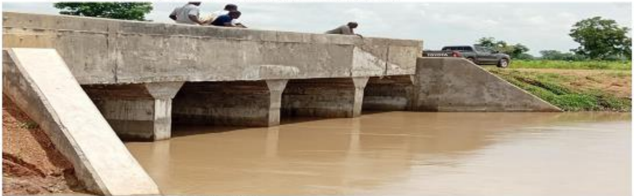
U CULVERT AND BRIDGE AT GBANGBANPONG-NAKPEL FEEDER ROAD
