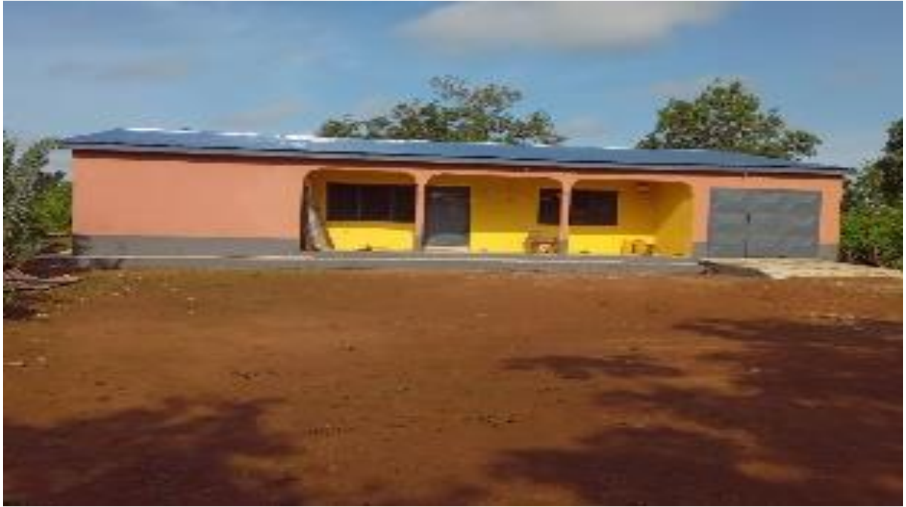
Rehabilitated 1NO. Semi-detached District Education Director's Quarters.
