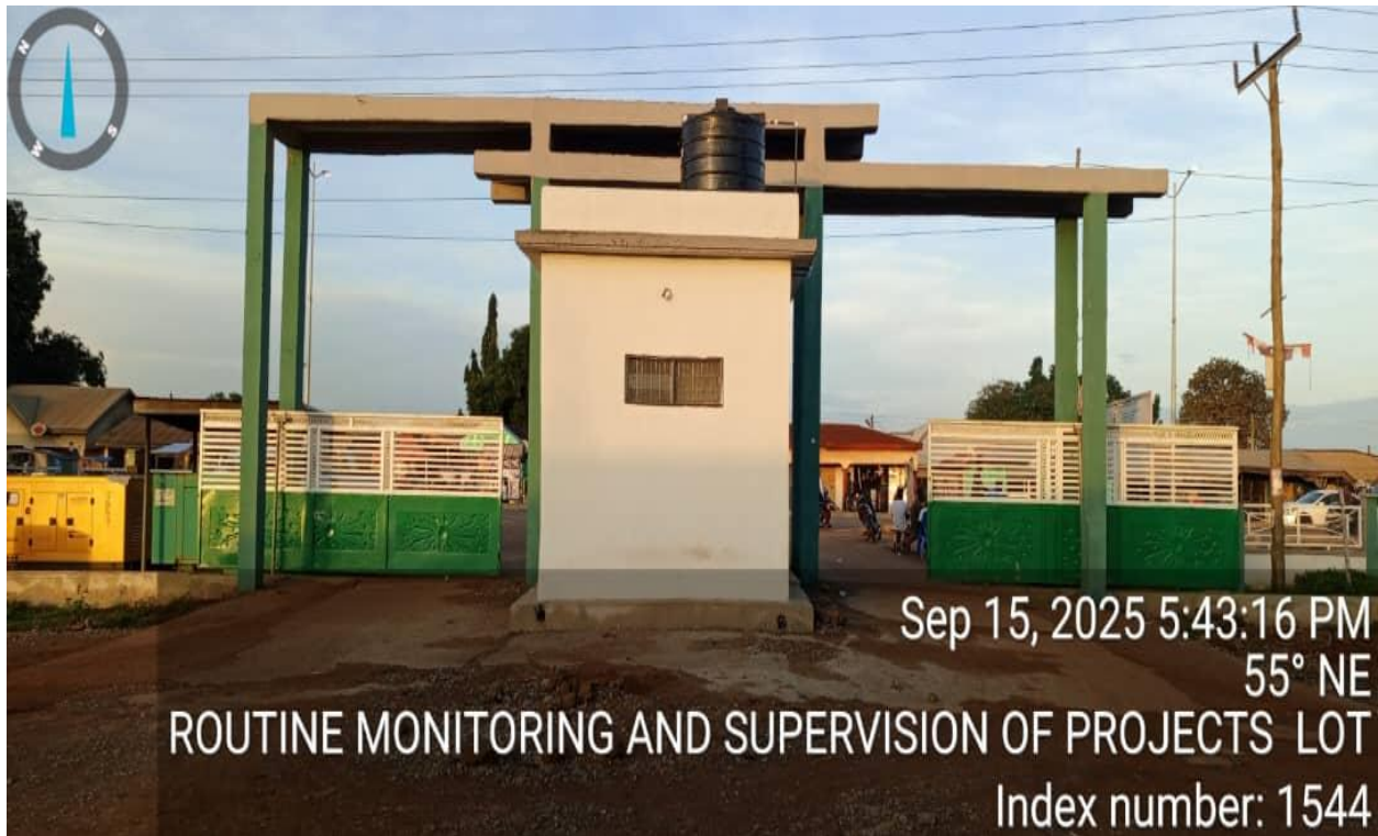
Constructed Bimbilla Hospital Wall, Dual entrance, security post and 2No. Exit gates
