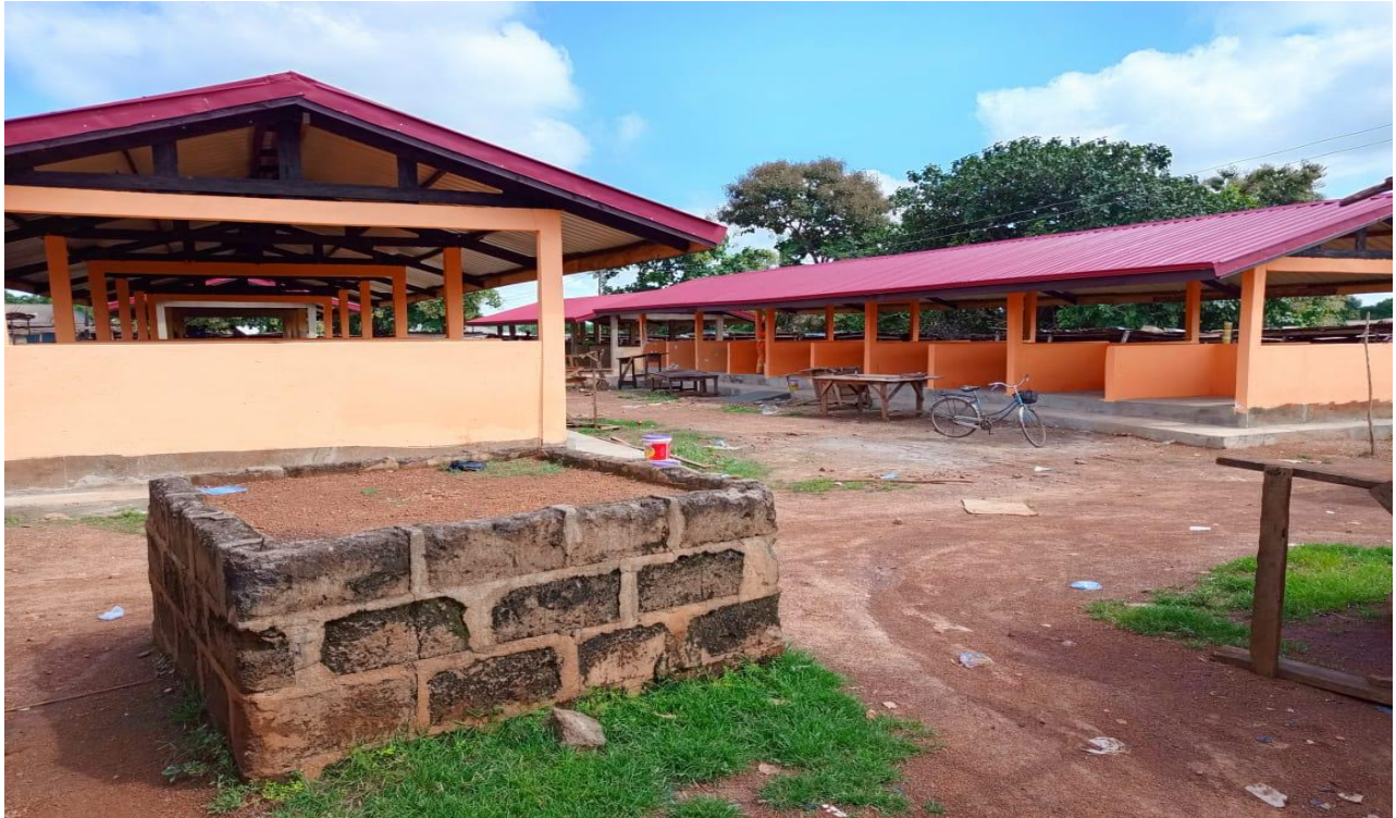
Rehabilitated 2No. 20-unit open market sheds at Chamba
