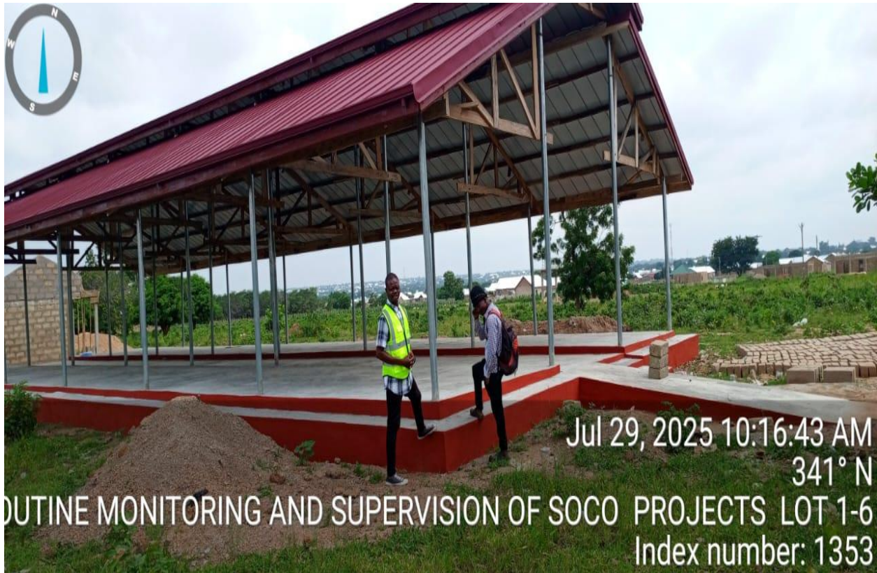
Constructed 1No. 14-unit open market shed at Bimbilla Yam Market
