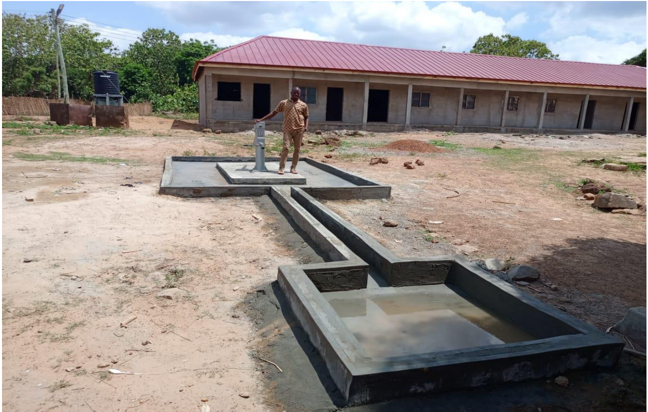
Drilled and installed 1 Borehole at Dipah
