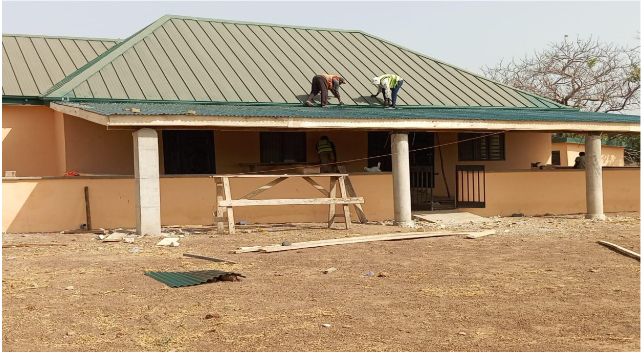
Nyingali CHPS Compound with Nurses Accommodation
