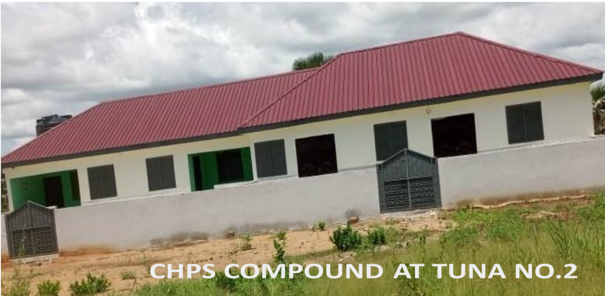
Fig.2 CHPS COMPOUND AT TUNA NO.2
