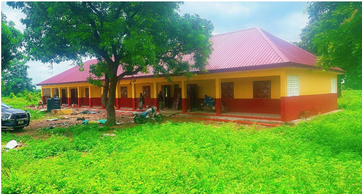
3-unit classroom block at Kuba
