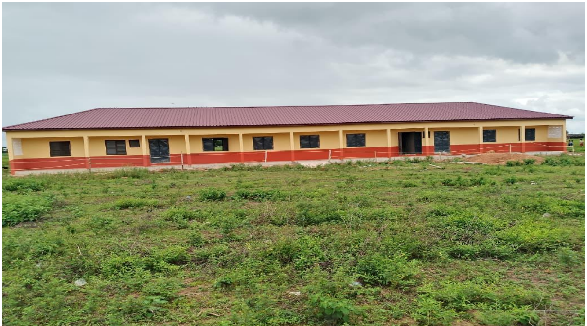
3unit classroom block at Tuni
