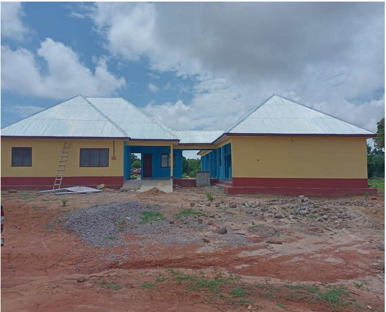
CHPS Compound at Dabari
