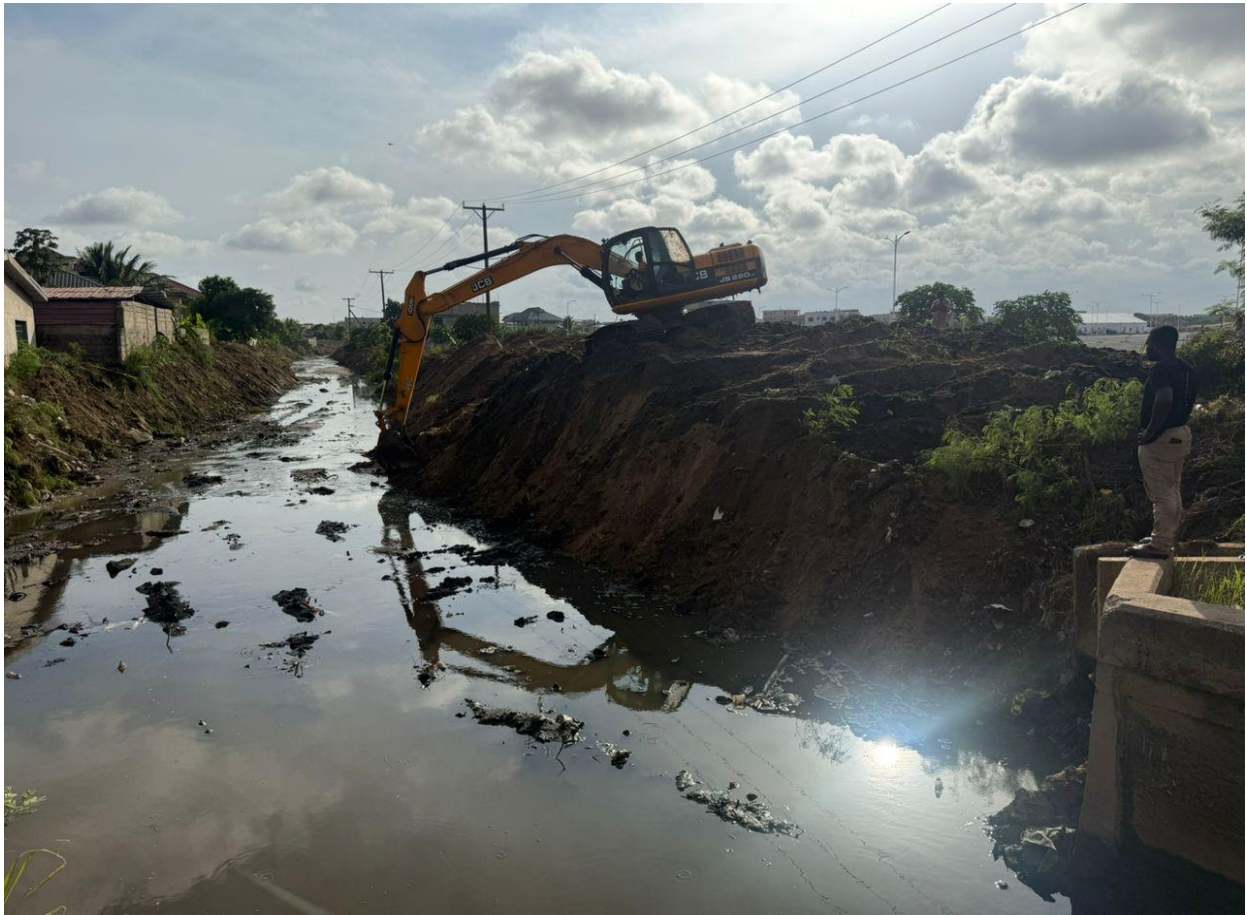
Storm Drains dredged at Teshie Bush road.
