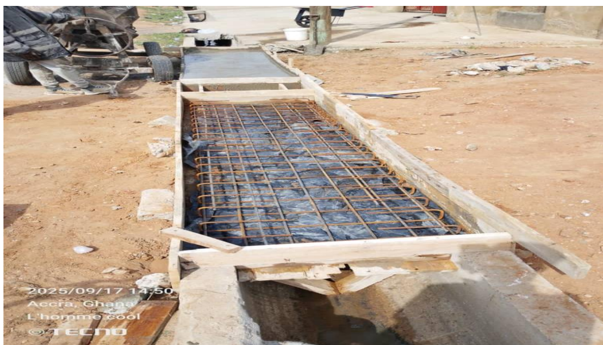
Constructed Septic tank at Dar-Es Salaam Basic school
