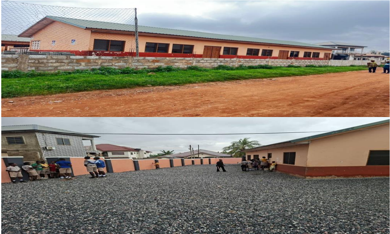
Constructed 1No. Fence Wall with Gate at Atiwoto MA School
