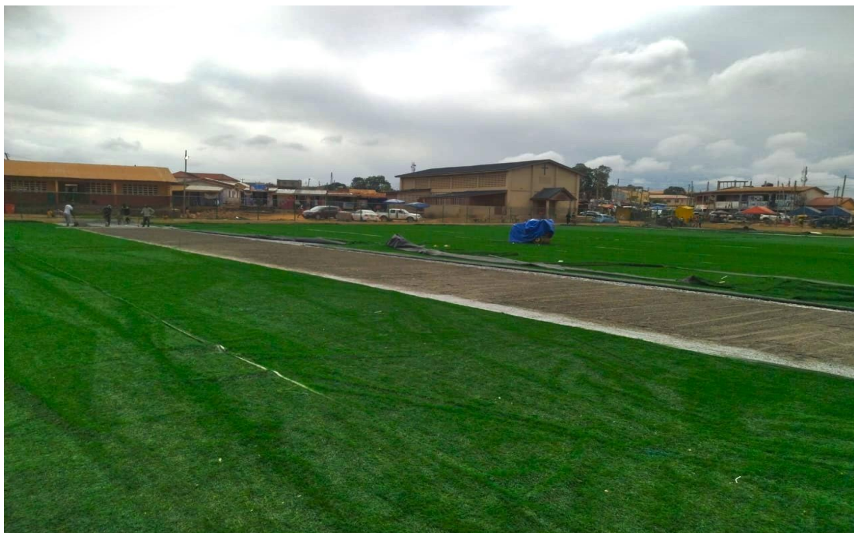
Construction of 1No Astroturf at Ofankor MA Basic School
