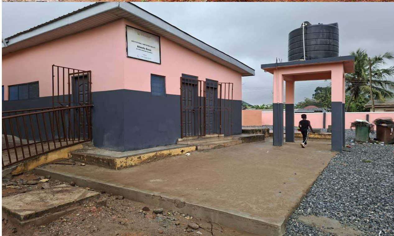
Renovated 1No. 17 Seater WC Toilet at Atiwoto MA Basic School
