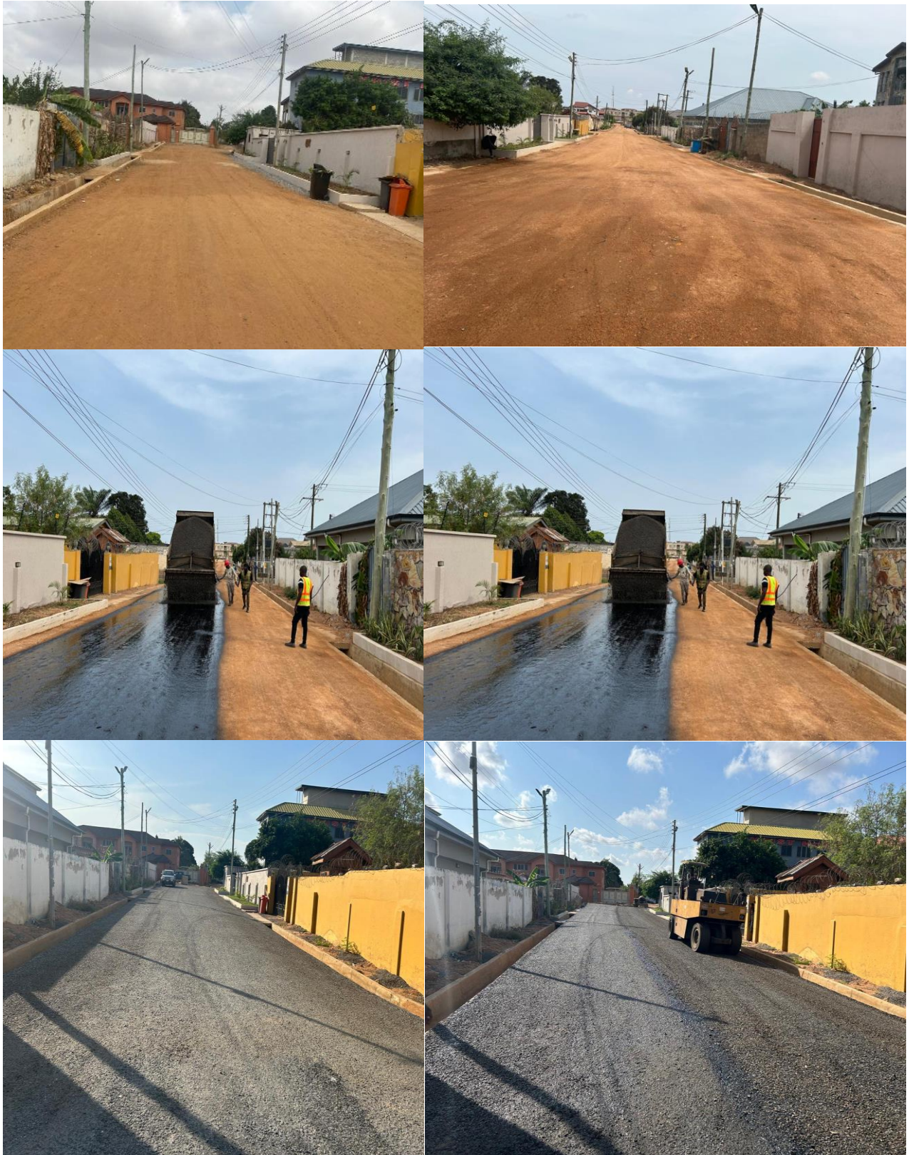
Rehabilitated Nummo Ntkeh Street (0.3km) Road
