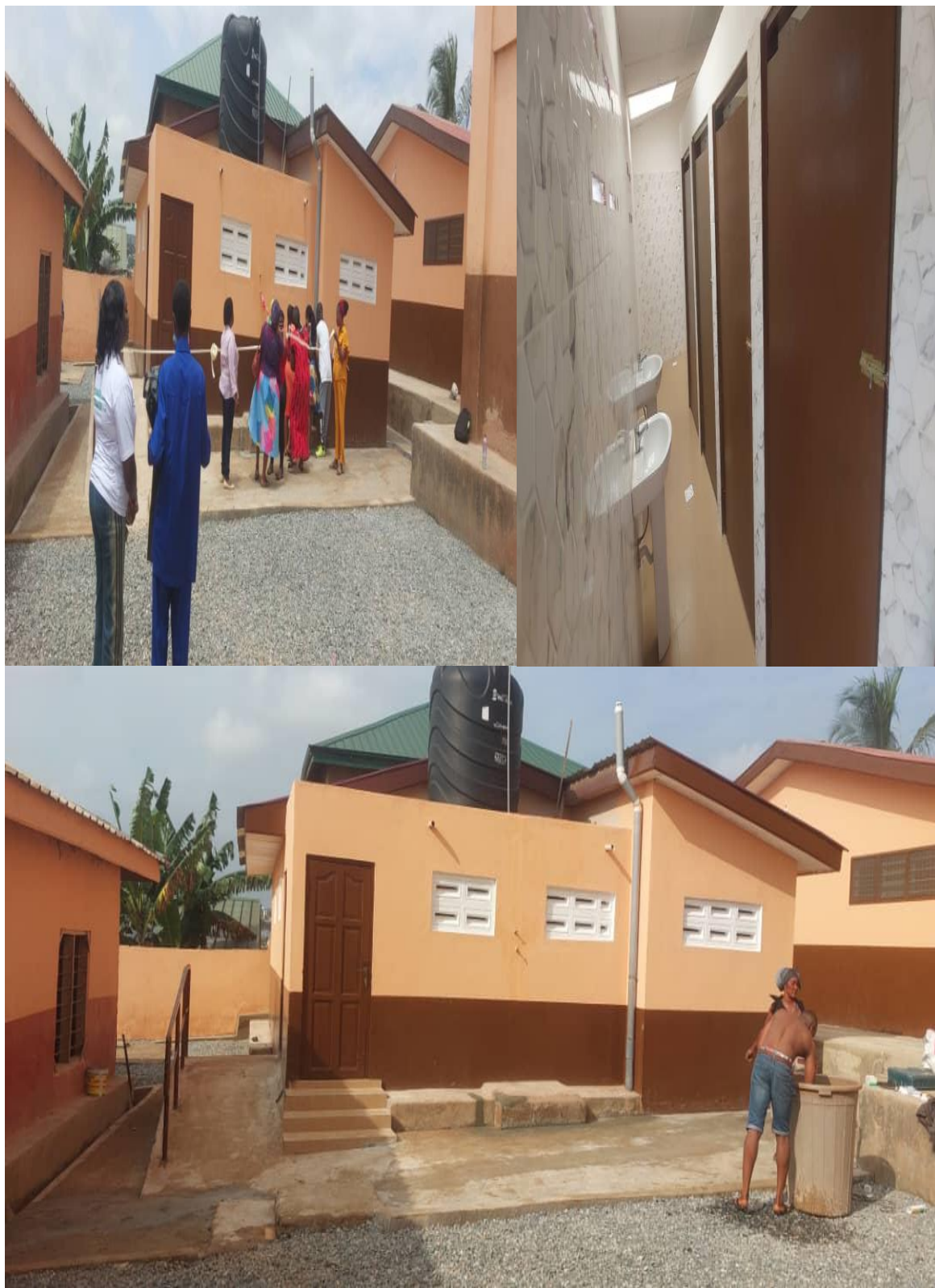
Completed 1No. 16 Seater WC Toilet at Omanjor MA Cluster of Schools
