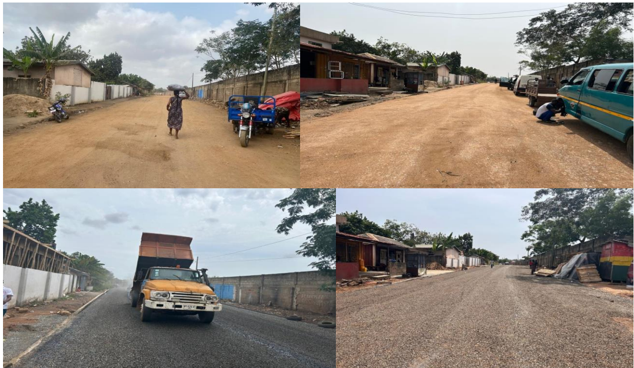
Rehabilitated Liberation Street (0.2km) Road
