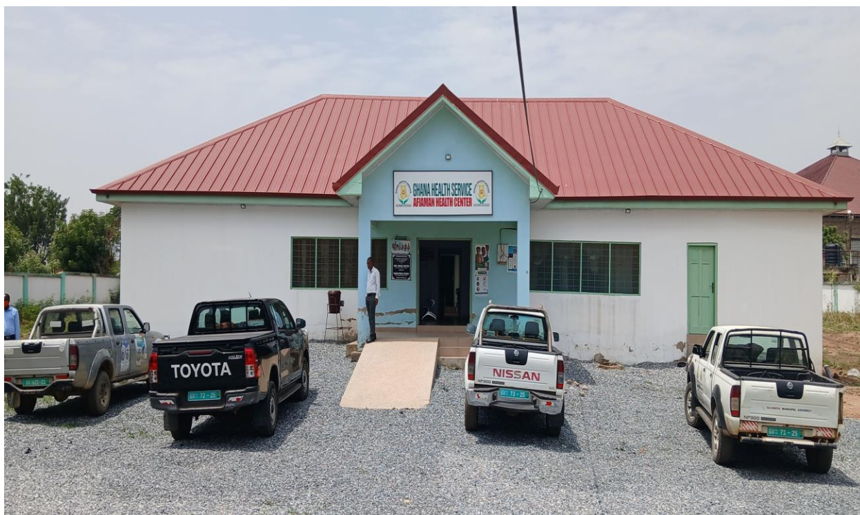
Completed 1No CHPS Compound at Afiaman
