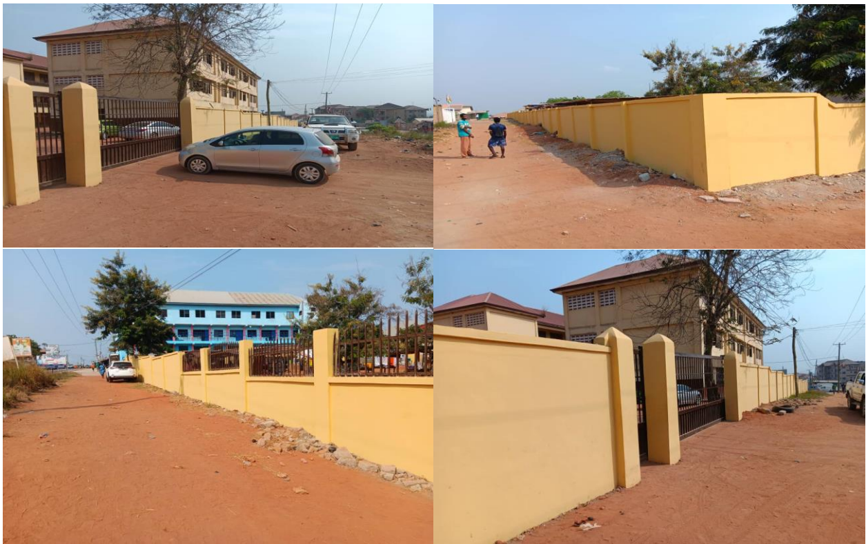
Constructed 1No. Fence Wall with Gate at Asofan Basic School
