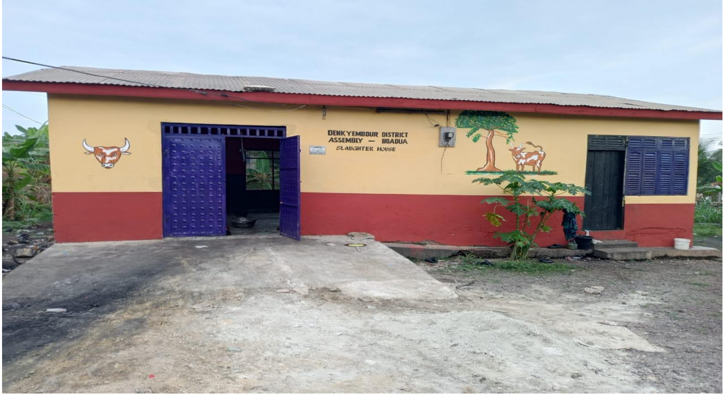
Renovation of slaughter house at Boadua
