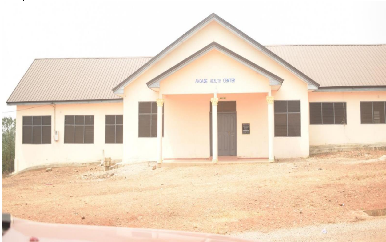
Completed 1No. Health Centre at Akoase
