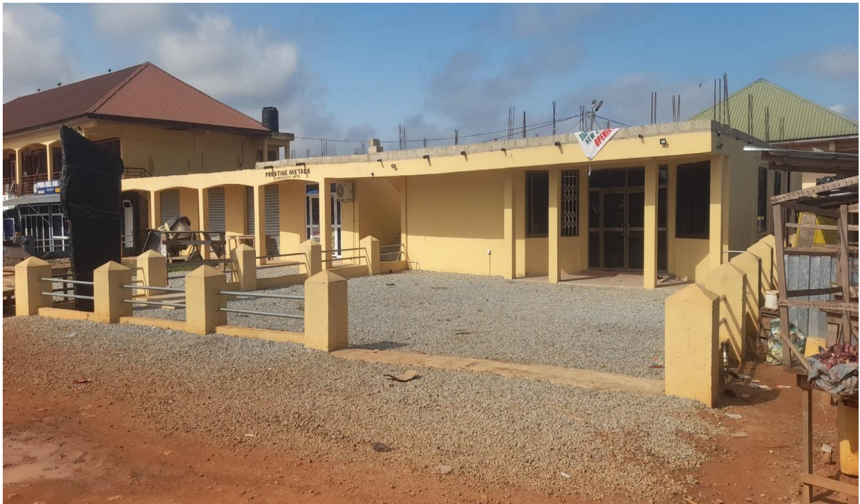
Completed 1 NO. 8-Lockable Stores and Banking Hall Complex at New Abirem
