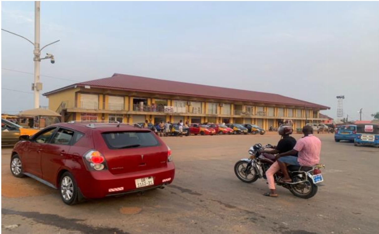
Completed 64 Lockable Stores at New Abirem
