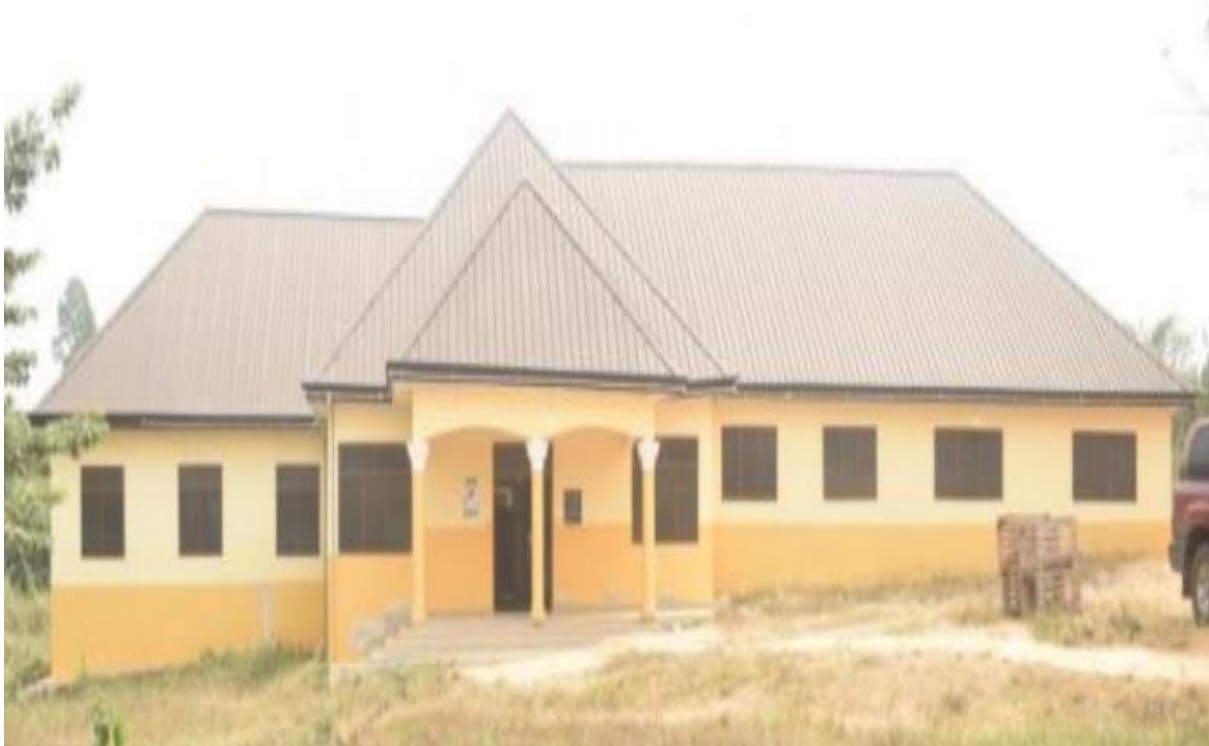
Completed 1No. Health Centre at Pankese
