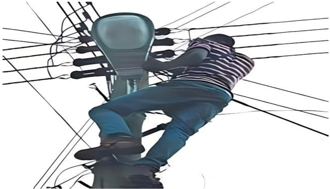
Rehabilitation of Streetlights in the District
