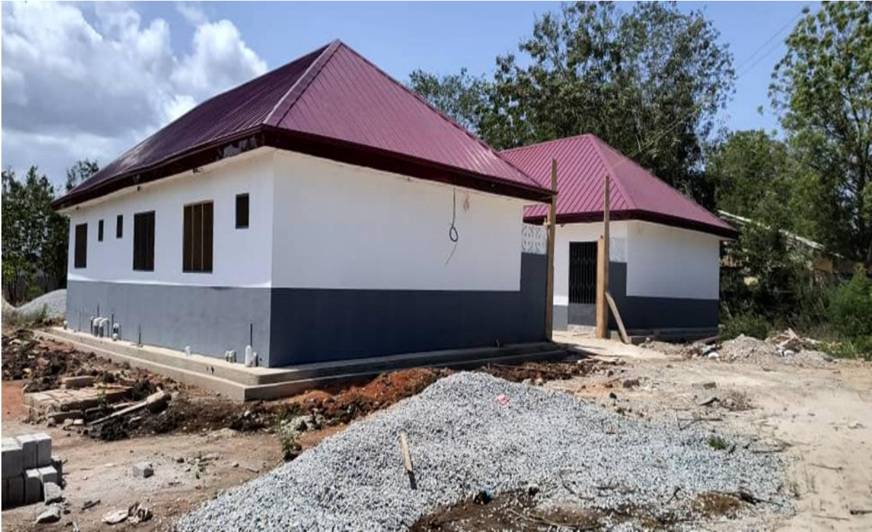
Figure 5: Completed a 1No 6unit Teachers' quarters at Apam
