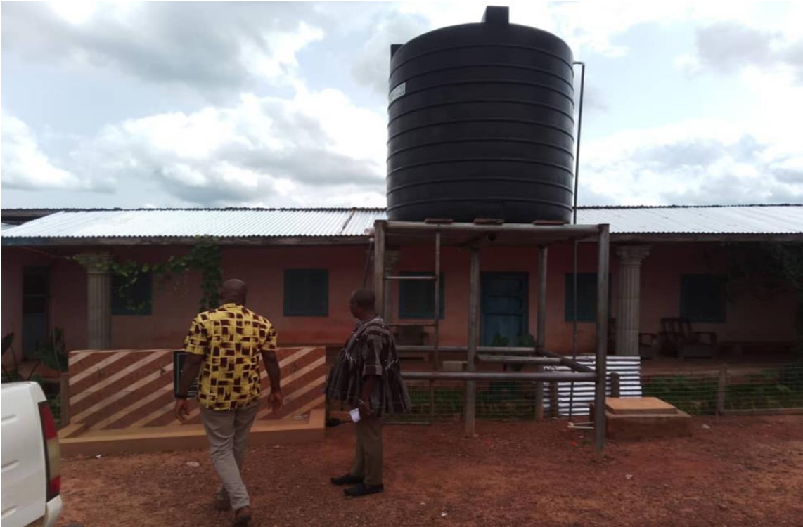
Figure 4: Completed a mechanized Bole hole with poly tank and electricity connection at Gomoa Ayanful
