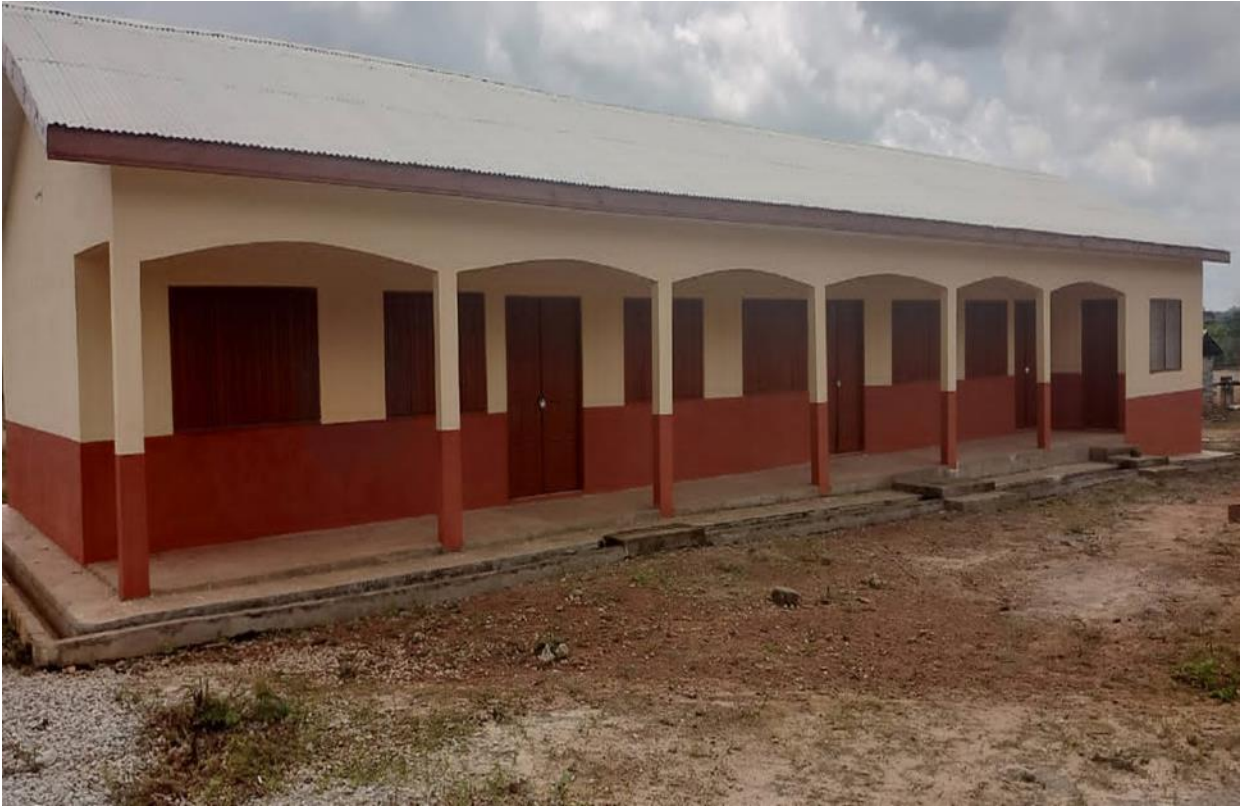
Figure 2: Constructed 1no. 3unit classroom block with store and Staff common room at Appiakrom Debiso
