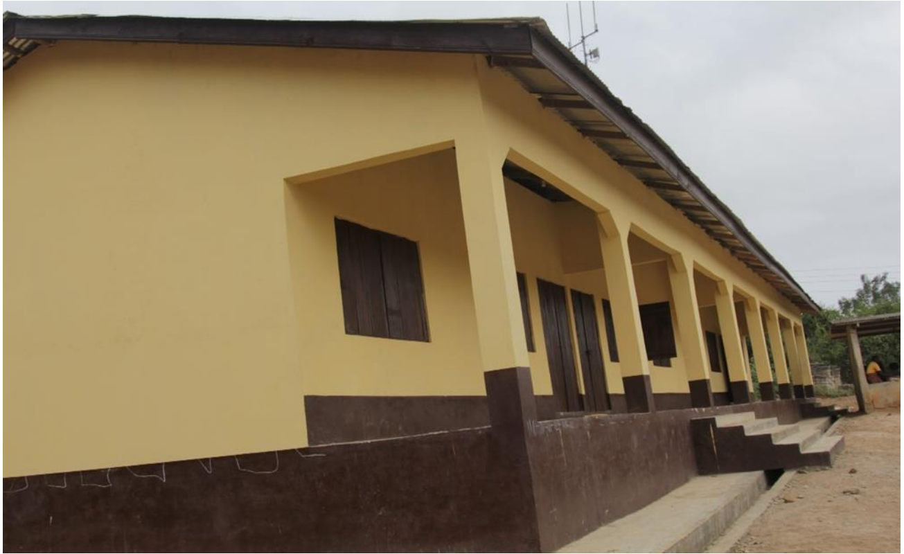
Figure 1: Completed 1 No 3-Unit Classroom block with KVIP at Gomoa Obiri
