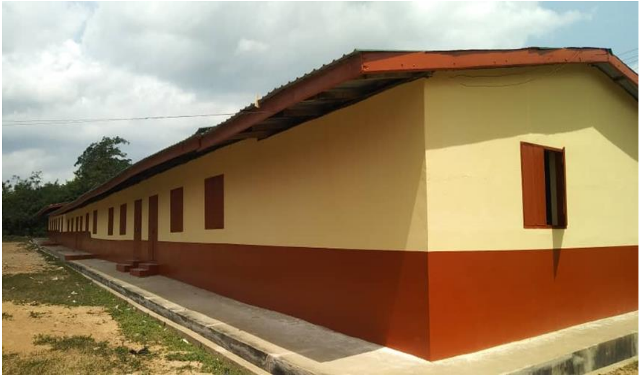
COMPLETED THE REHABILITATION OF SIX (6) UNIT CLASSROOM BLOCK AT DEHIA -DACF
