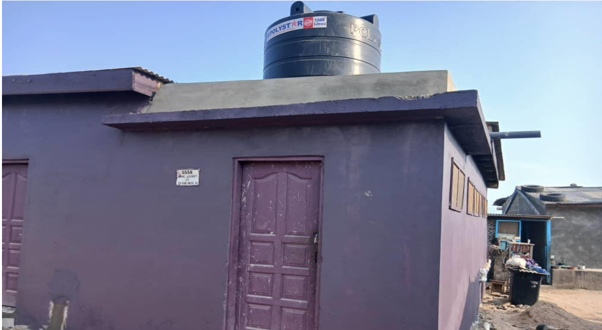
COMPLETED 8-SEATER W/C AND 4- UNIT SHOWER AT AMANFUL -DACF
