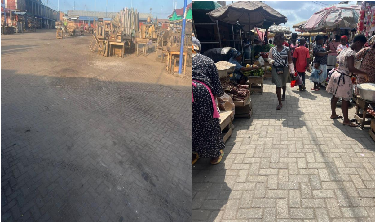
Fig. 7 – PAVEMENT WORKS AT KASOA NEW MARKET
