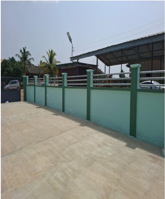
Fig. 11 – 6-UNIT CLASSROOM BLOCK AT NAHADATU SCHOOL
