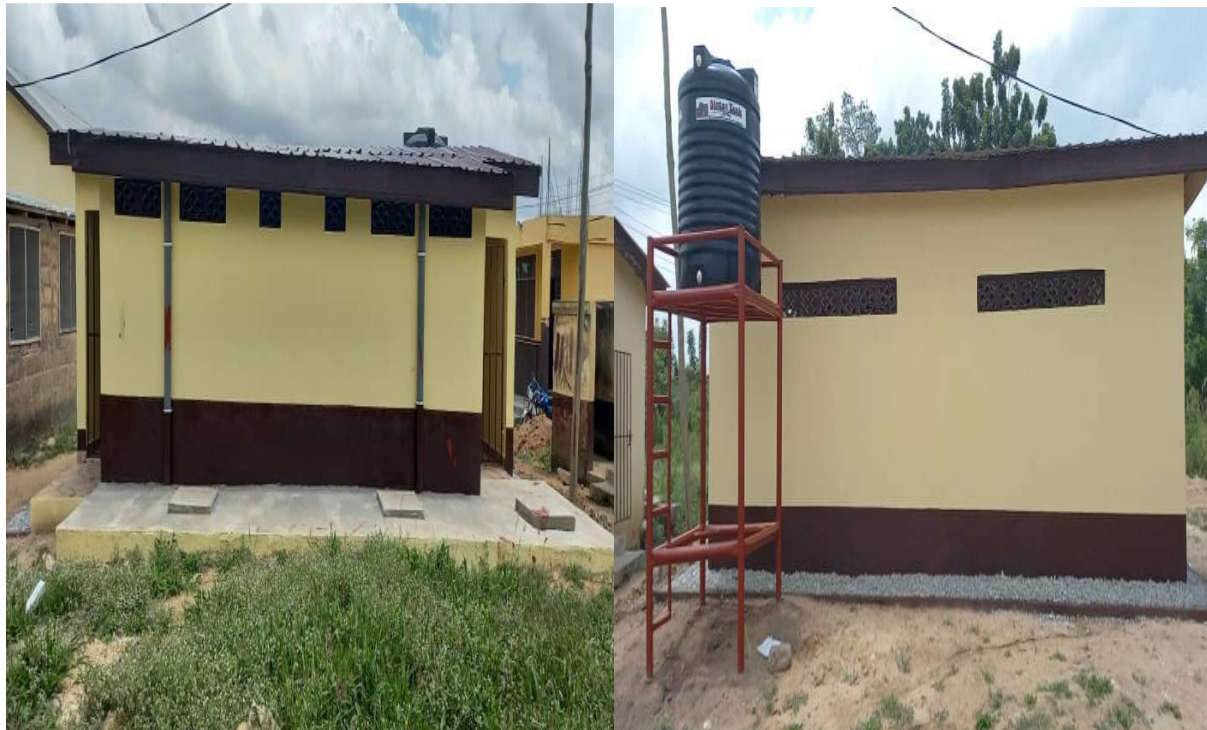
Fig. 8 – 6-SEATER WC TOILET FACILITY AT AKWELEY
