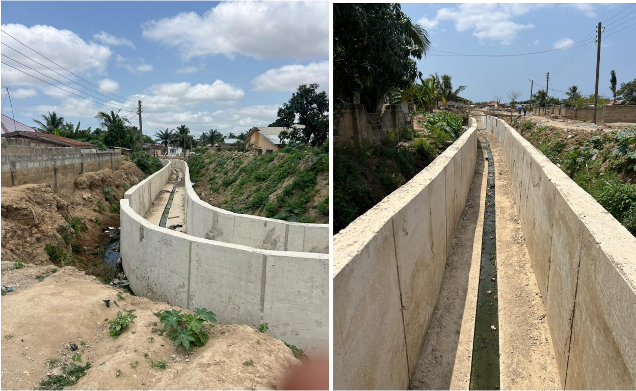
Fig. 4 – BOX CULVERT FROM WALANTU TO KASOA
