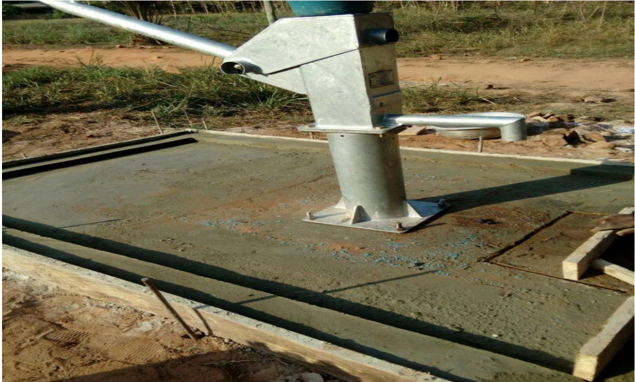
1 no. hand pump borehole constructed at Nuanua Krobo.
