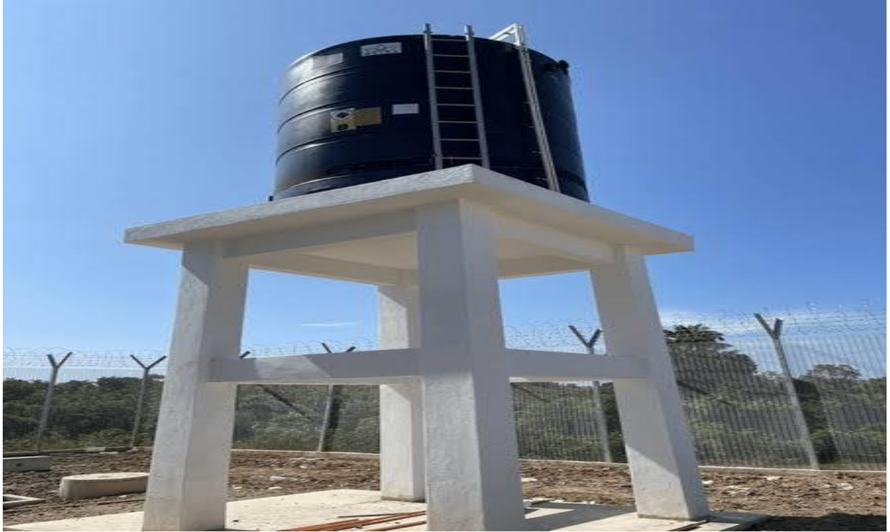
1 no. mechanised borehole with overhead tank constructed at Assin Akomanim.
