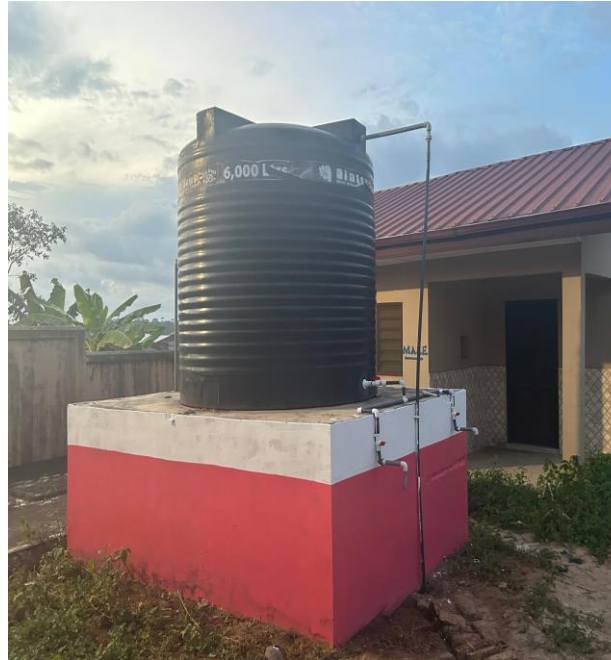
Drilled and Mechanized 7 No. Boreholes with over-head polytanks
