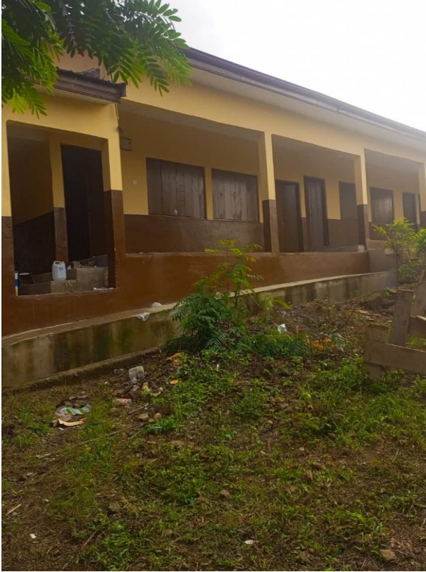
Completed the Construction of 1 No. 3 unit classroom block with Office, computer lab and washroom at Ninta Methodist school
