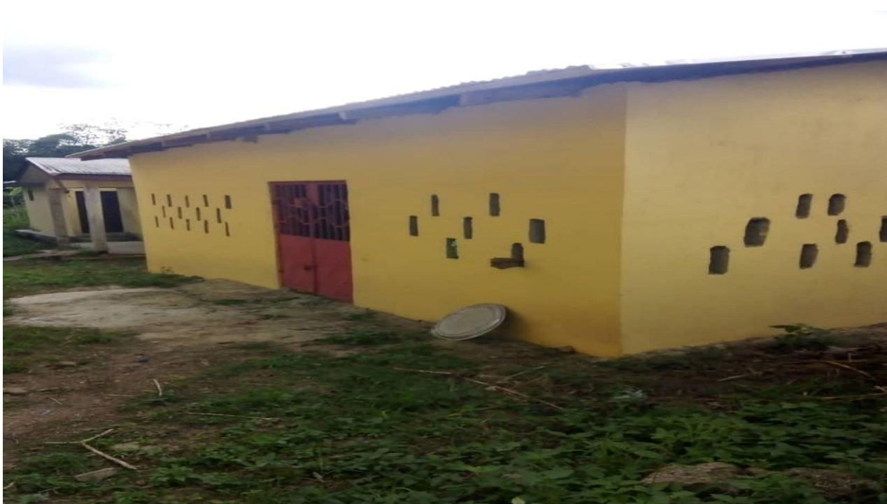
1. Constructed Animal pound to impound stray animals for revenue generating
