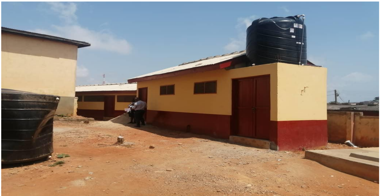
Constructed 1 No. 7 seater and Construction of 1No. 5 seater Institutional Latrine at Moree.
