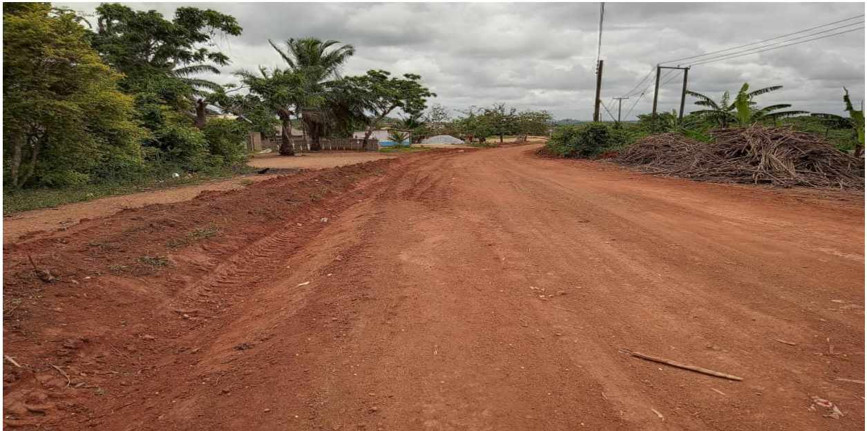
Reshaped Putubiw - Apewosika Feeder Road
