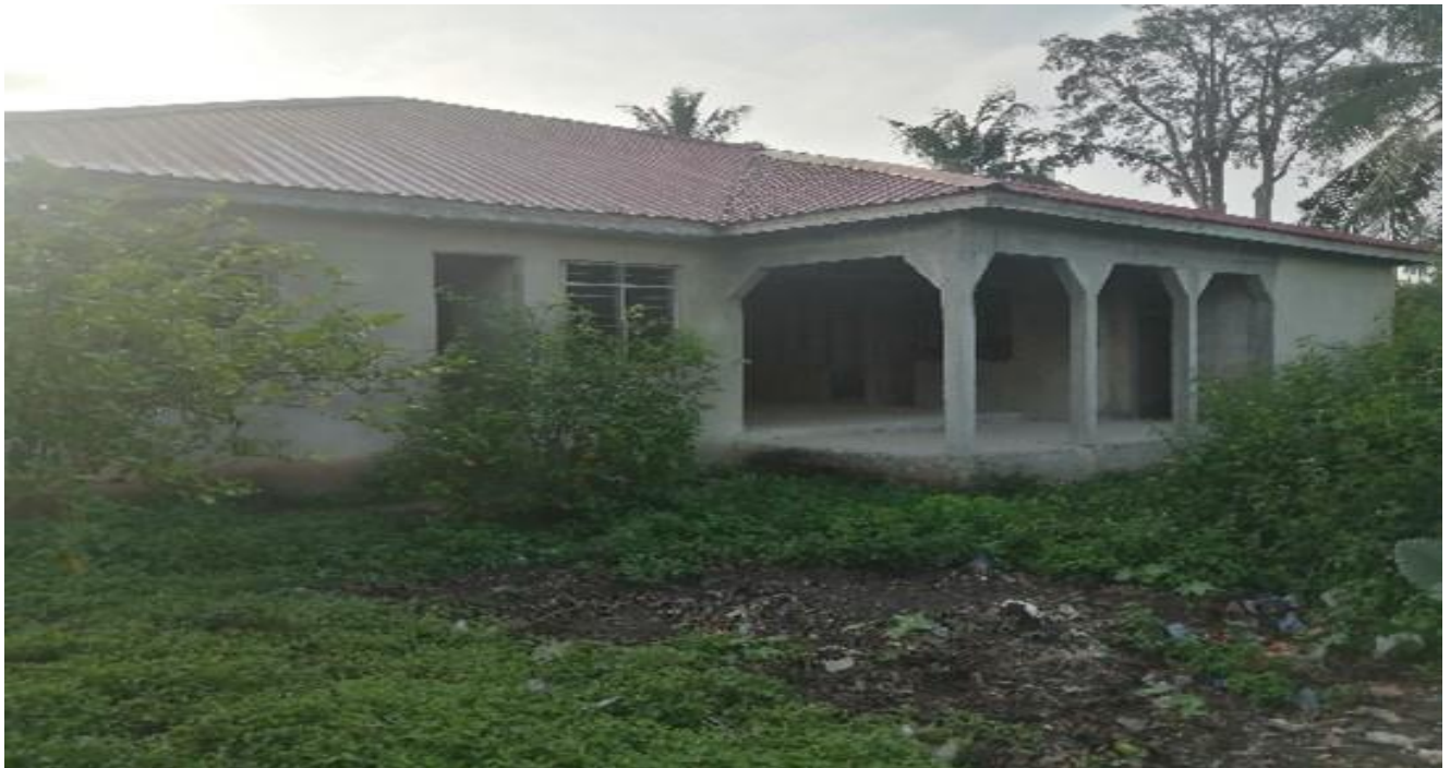
Completed 1No. CHPS Compound at Abaka
