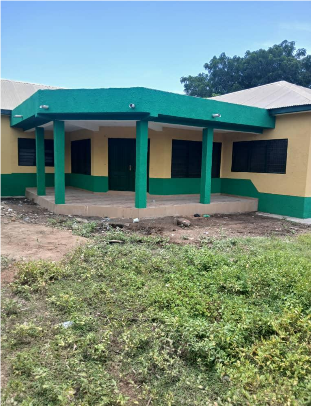
Completed the department of Agriculture office complex
