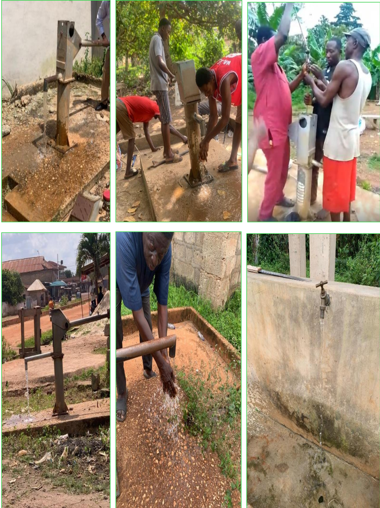
Picture 4: Rehabilitated 20No. Boreholes in Berekum Municipality.
