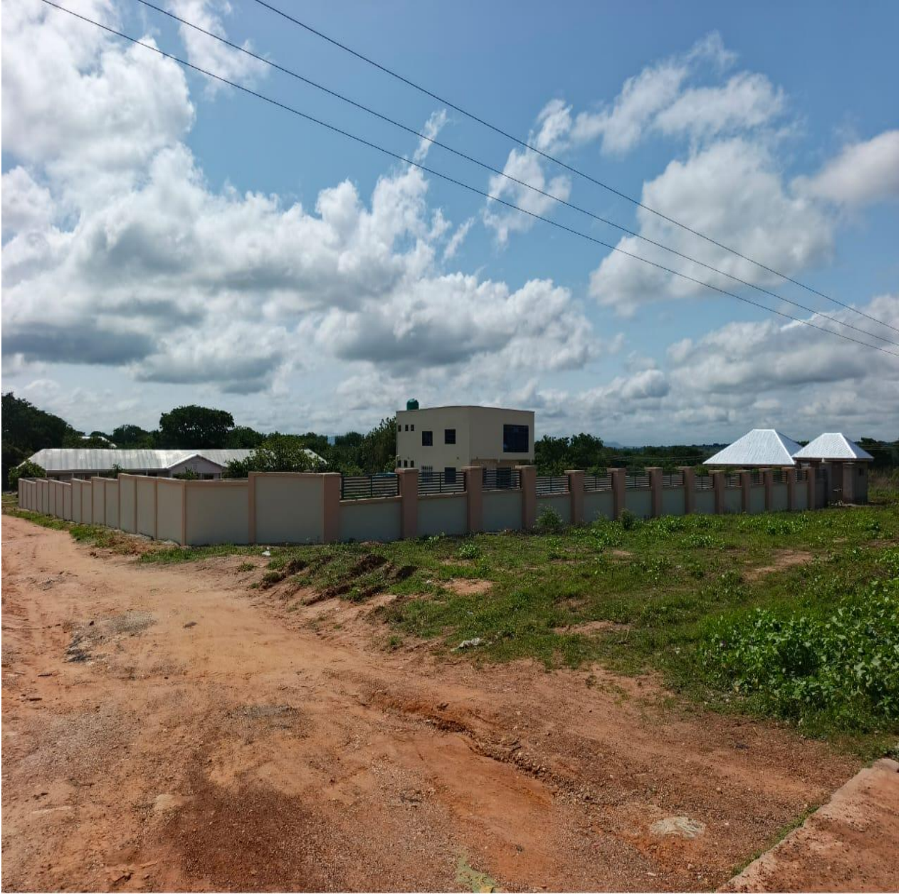
Picture 1: Completed and furnished a District Police Headquarters at Banda Ahenkro
