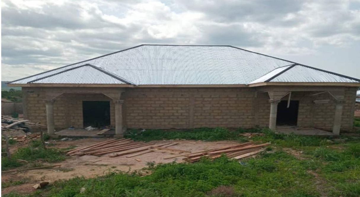
Picture 4: Constructed 1No. Warehouse at Bongase Fish Market
