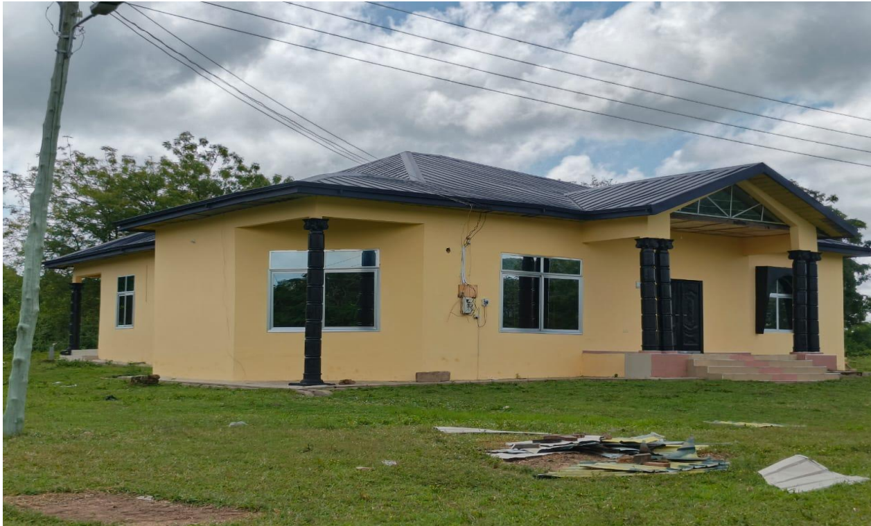
Picture 3: Renovated and Furnished the DCE's Bungalow at Banda Ahenkro
