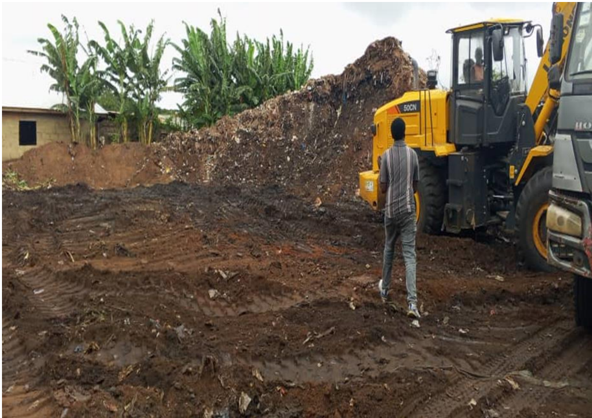
AFTER EVACUATION OF REFUSE DUMP AT TUOBODOM ZONGO COMPLETED
