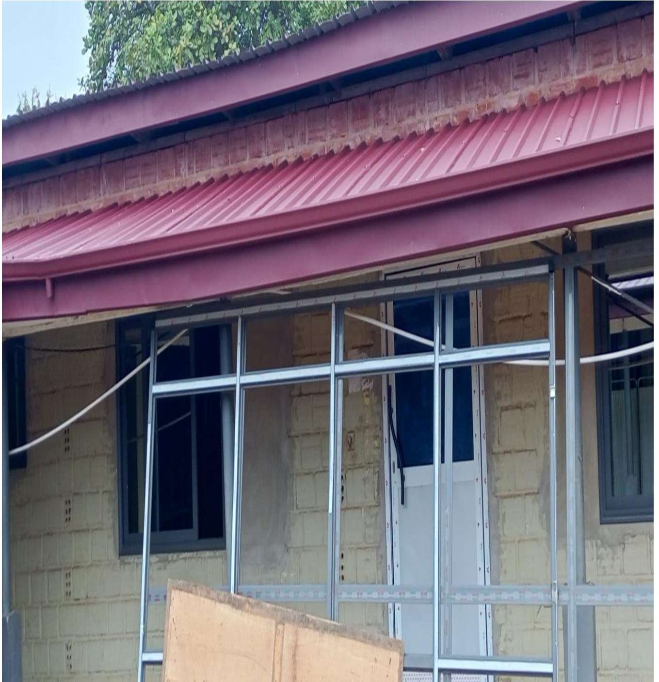
RE-ROOFING OF POLY-CLINIC AT TUOBODOM COMPLETED
