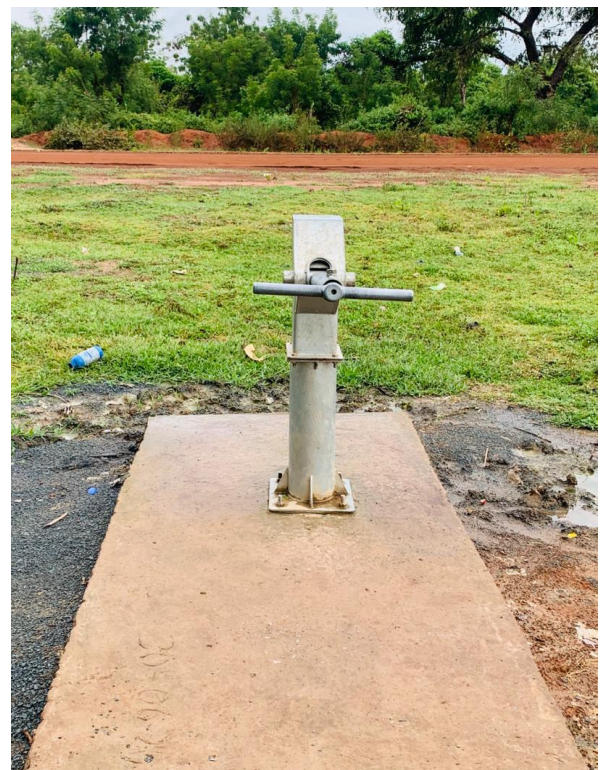
Constructed 2 No. Boreholes with IGF (1 with a Hand pump, and one mechanised)
