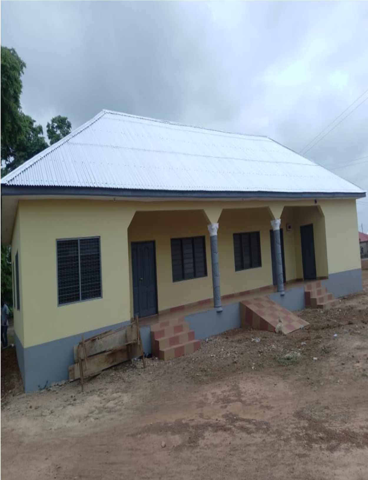
Completed 12 Bed Ward at Parambo (MPCF)
