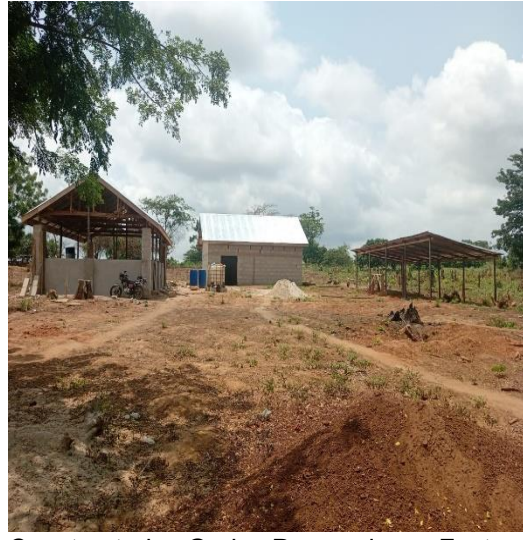
Constructed Gari Processing Factory at Johnkrom (Remark: 85% completed)
