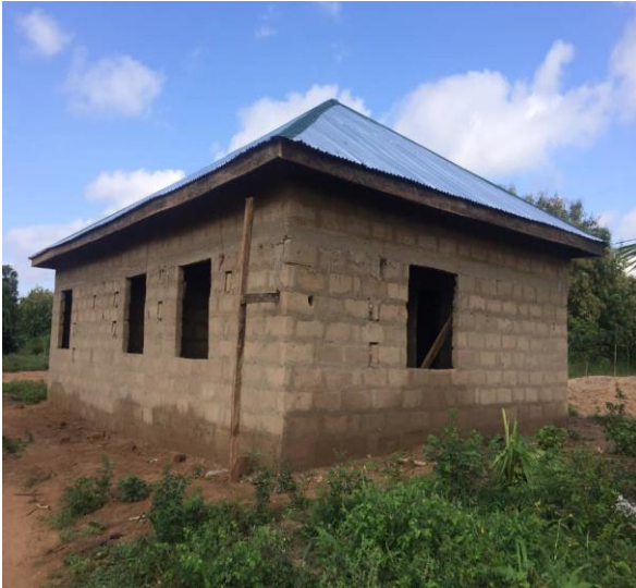
Constructed Teachers quarters at Kwafre (Remark: 60% completed)
