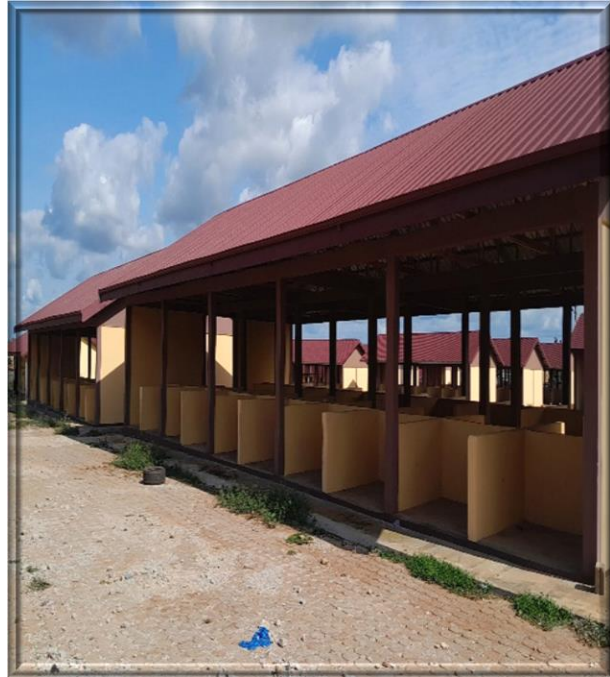
(Remark: Roofing, painting and floor works done in 2025)
