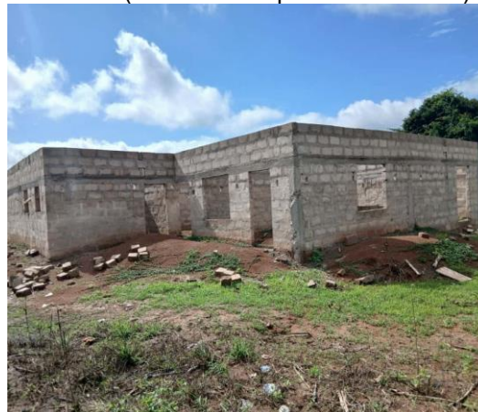
Constructed 1No. CHPS compound at Kyekyewere (Remark: 40% completed)
