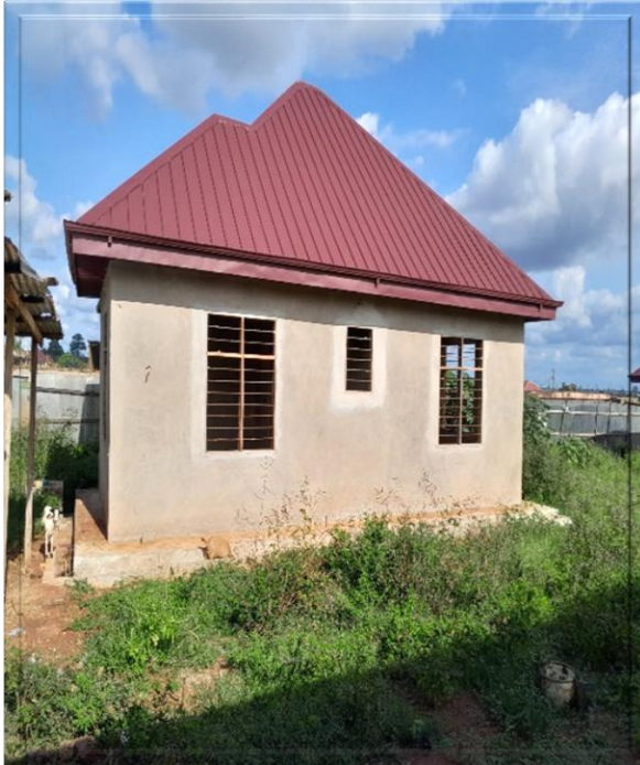
(Remark: Roofing and Plastering works done for 2025)
