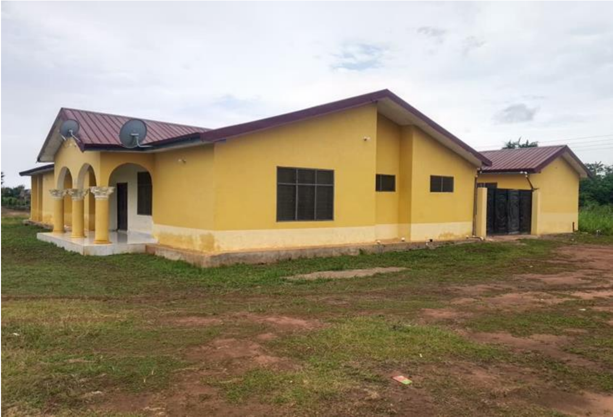
6-Bedroom DCE Residence at Busunya
