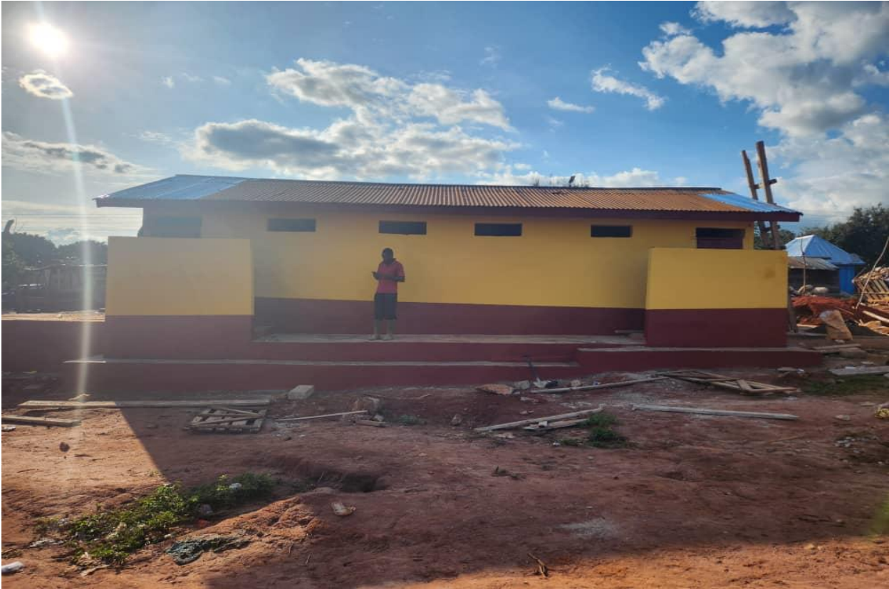
20-Seater KVIP Toilet at Busunya
