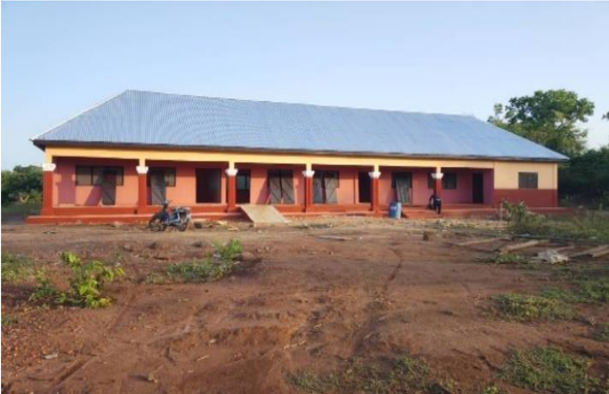
Completion of 1No. 3-Unit Classroom at SDA Primary, Kintampo
